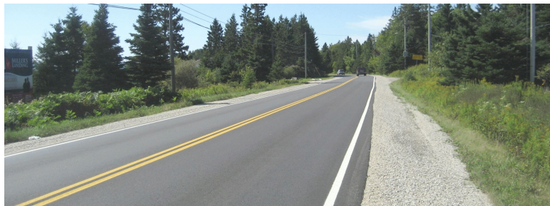
Photo 2-4 - Looking west on Trunk 3 towards Hubbards from the proposed intersection location for connector Options 2 and 3A. Visibility is adequate for the posted 70 km/h speed limit.
