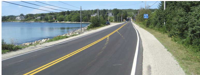
Photo 2-2 - Looking west on Trunk 3 towards Hubbards from the proposed intersection location for Option 1 connector. Visibility is adequate for the posted 70 km/h speed limit.
