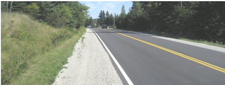
Photo 2-3 - Looking east on Trunk 3 towards Tantallon from the proposed intersection location for connector Options 2 and 3A. Visibility to the intersection may be marginal and must be considered during intersection design.
