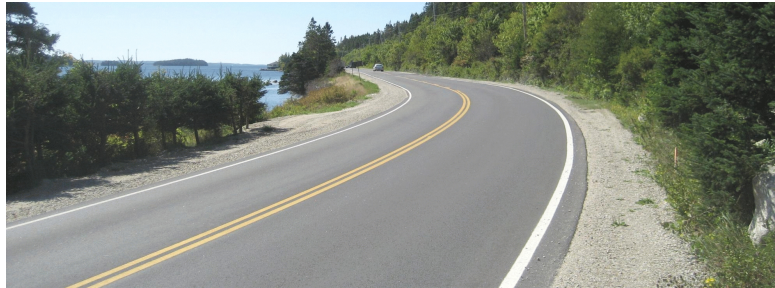
Photo 2-6 - Looking west on Trunk 3 towards Hubbards showing the character of Trunk 3 near the proposed Options 3B/C and Option 4 connector intersections.
