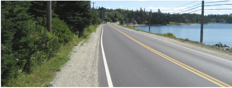
Photo 2-1 - Looking east on Trunk 3 towards Tantallon from the proposed intersection location for the Option 1 connector. Visibility is adequate for the posted 70 km/h speed limit.
