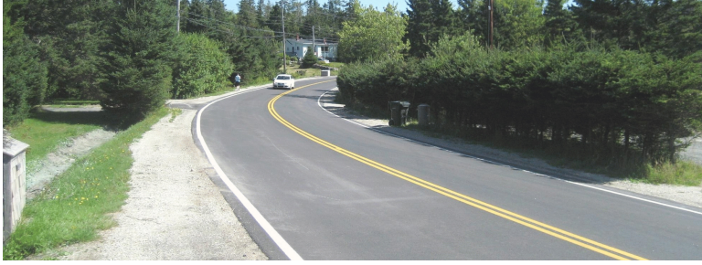
Photo 2-5 - Looking east on Trunk 3 towards Tantallon showing the character of Trunk 3 near the proposed Options 3B/C and Option 4 connector intersections.
