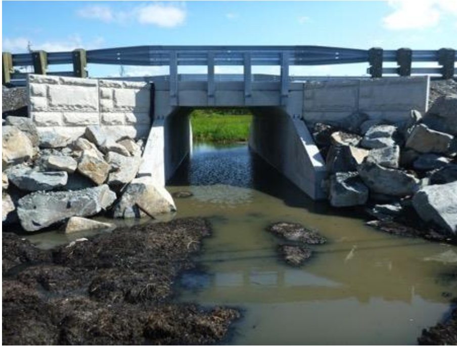
Figure 6 New tidal crossing installed July 2015. Photography by CBWES, July 16, 2015.
