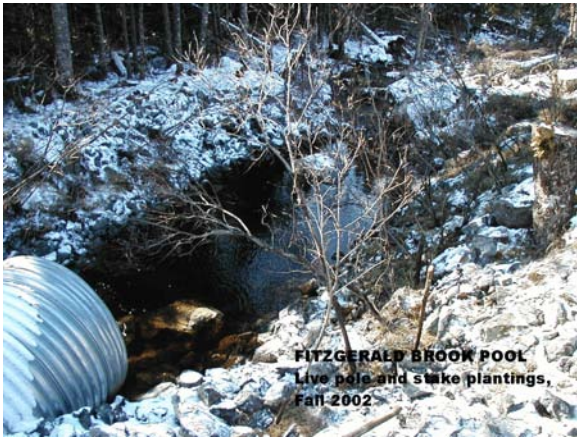
FITZGERALD BROOK PLUNGE POOL Live Willows from cuttings, Fall 2002, August 14, 2003
