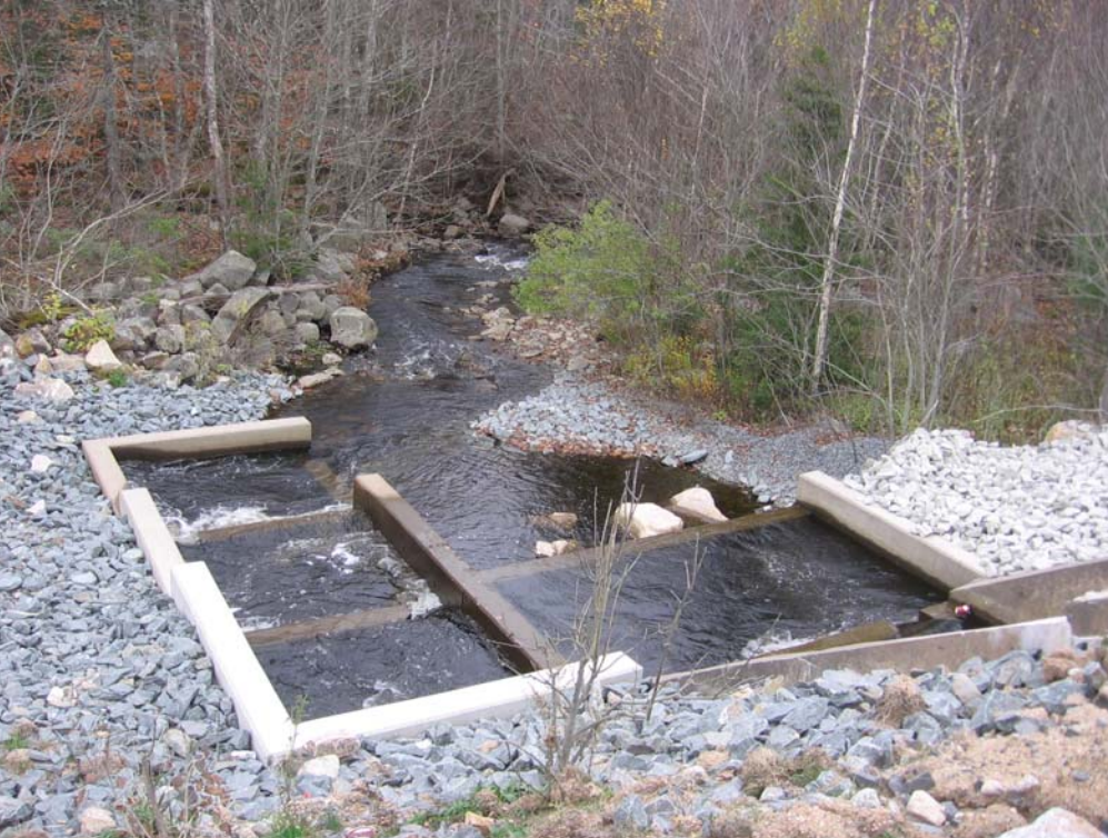
One year later – functioning well; high flow periods over the year had re-distributed the surge rock that buttressed the upper fishway box and formed the upper margin of the plunge pool (October 28, 2006)
