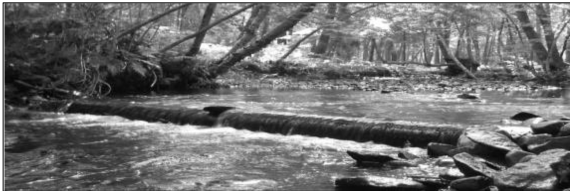
Figure 2. Digger Log installed by ACAP-Cape Breton on Cantley Creek August, 2004.
