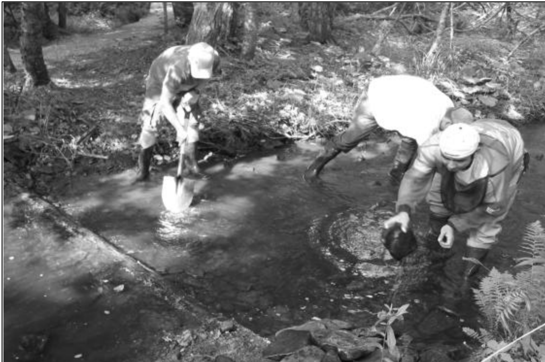
Figure 3. Installation of digger log by ACAP staff, August 2004.
