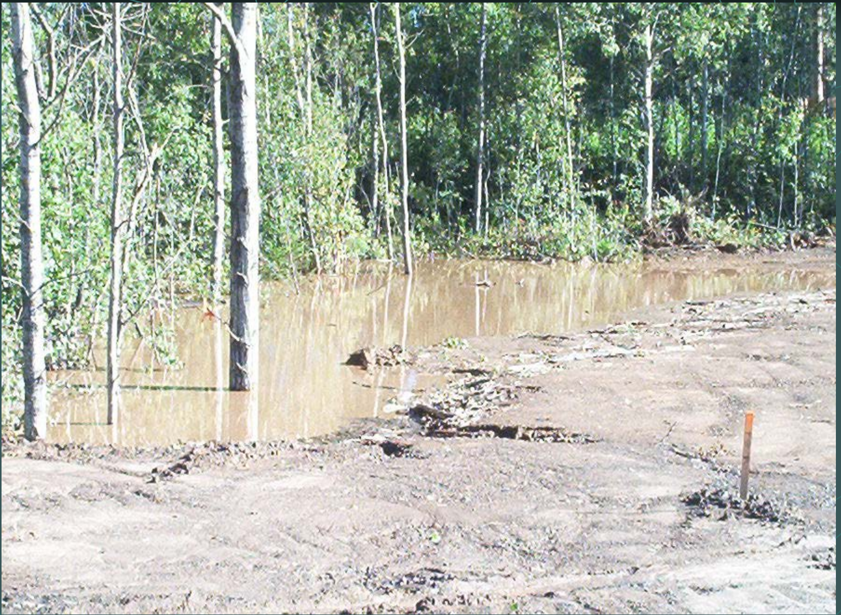
An “interim” sediment control pond
