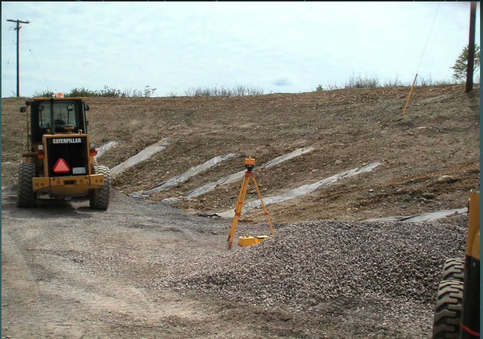
Relief Drains in Cut Slopes
