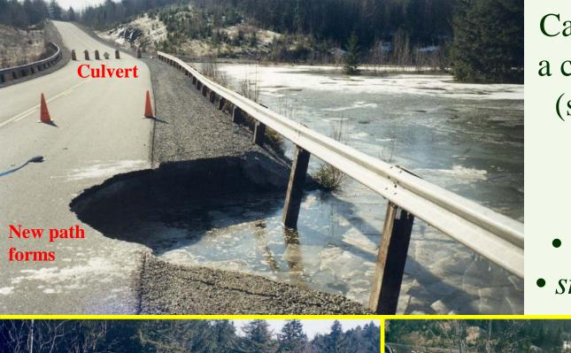
Catastrophic failure of a culvert on Route 374 (south of Stellarton) on April 2, 2003.
