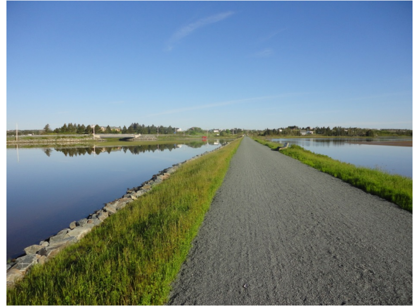
Finished Slopes Next Spring
