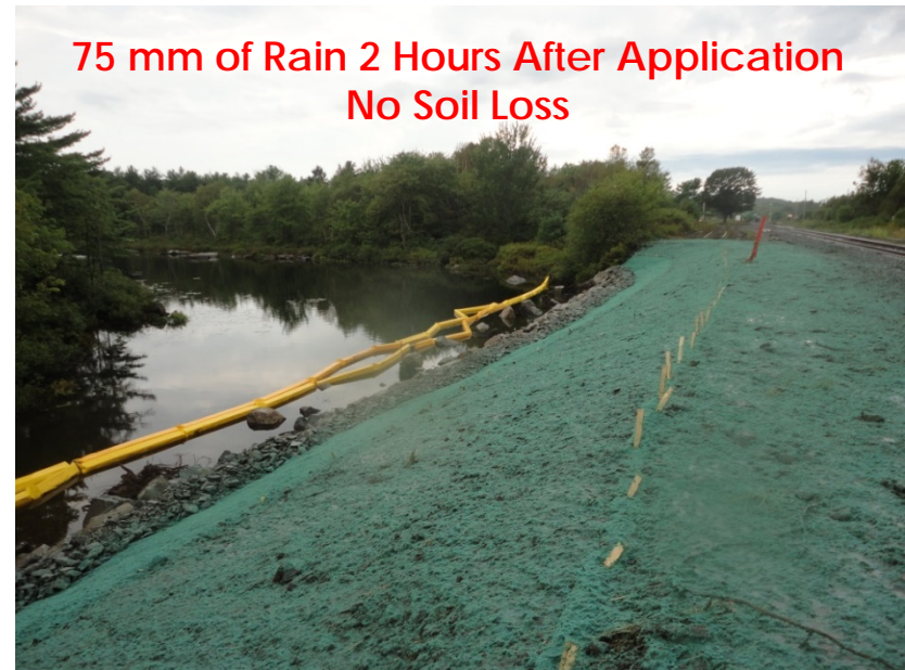
Permanent Stabilization of Slope
