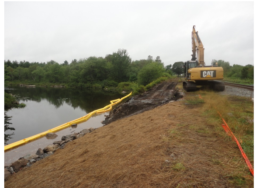
Cutting Back Existing 1.8 :1 Slope
