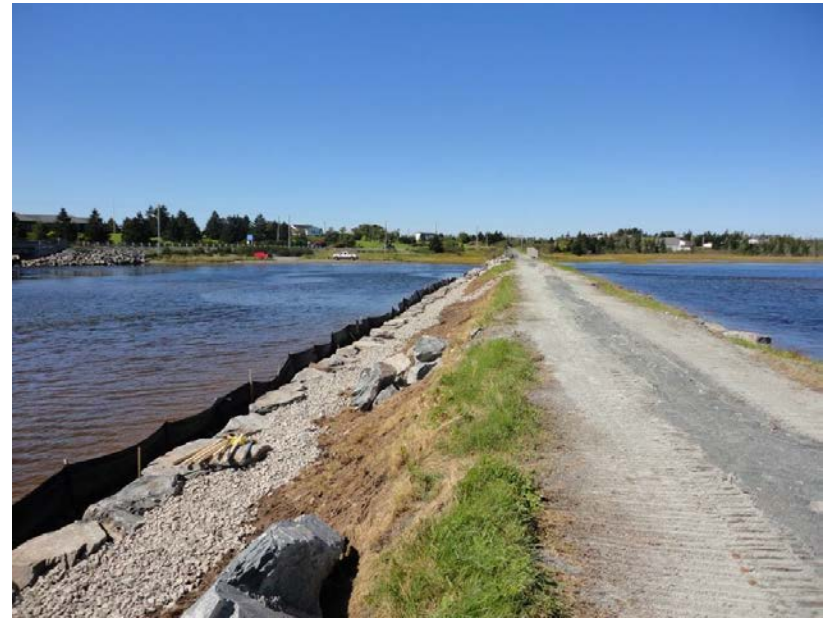
Armour Rock Placed to OHW
