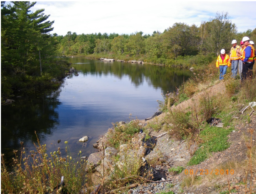
CN Embankment to be Cut Back
