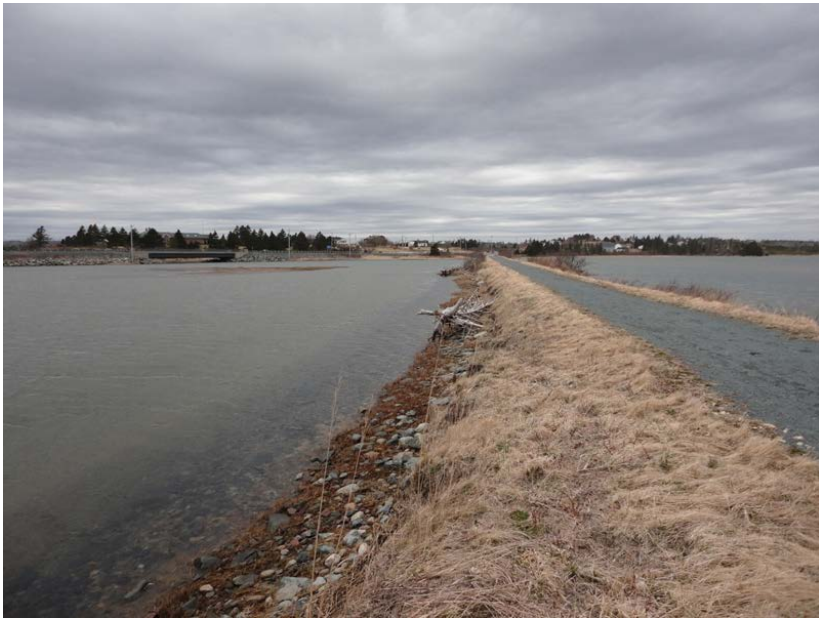
Slopes Eroded > 1:1
