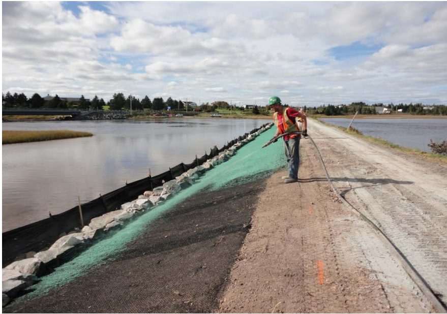
Hydraulic Mulch Applied to TRM
