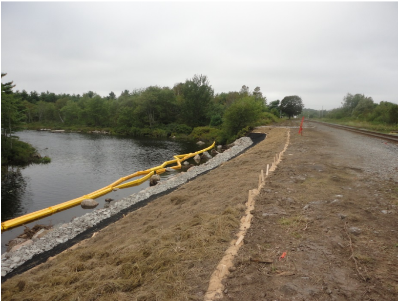
Temporary Stabilization of Slope
