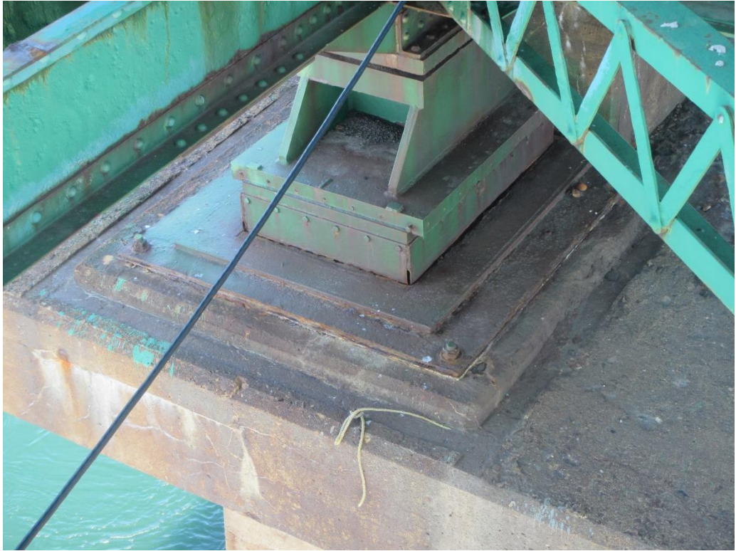
Figure 37: Pier 3 expansion bearing
