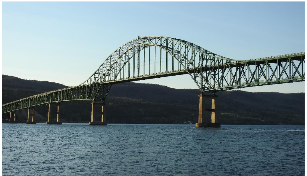
Figure 1: Seal Island Bridge south face (looking north)
