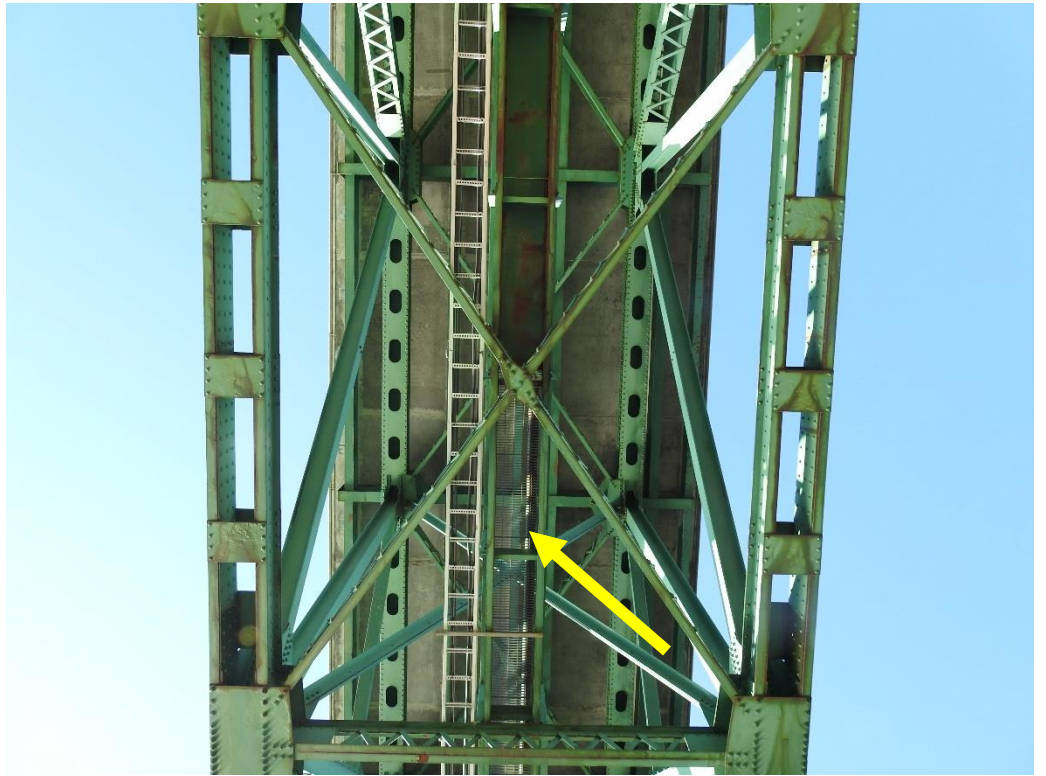
Figure 19: Underside view of approach truss showing longitudinal access catwalk
