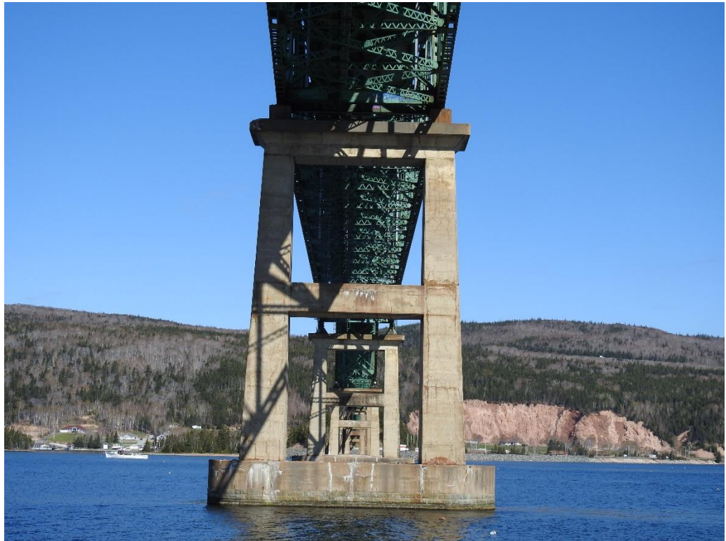
Figure 45: Typical substructure pier (Pier 7 shown)
