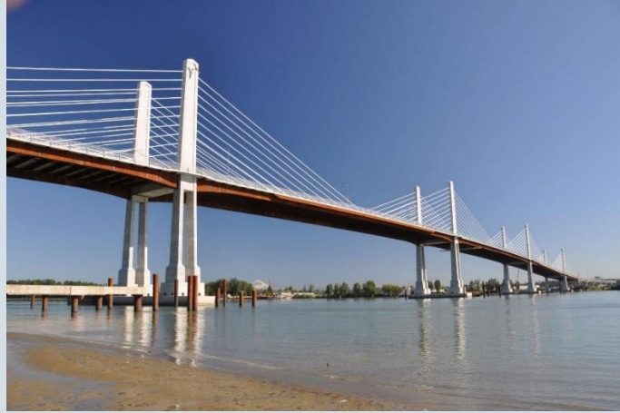
Golden Ears Bridge (Langley, BC, Canada):
