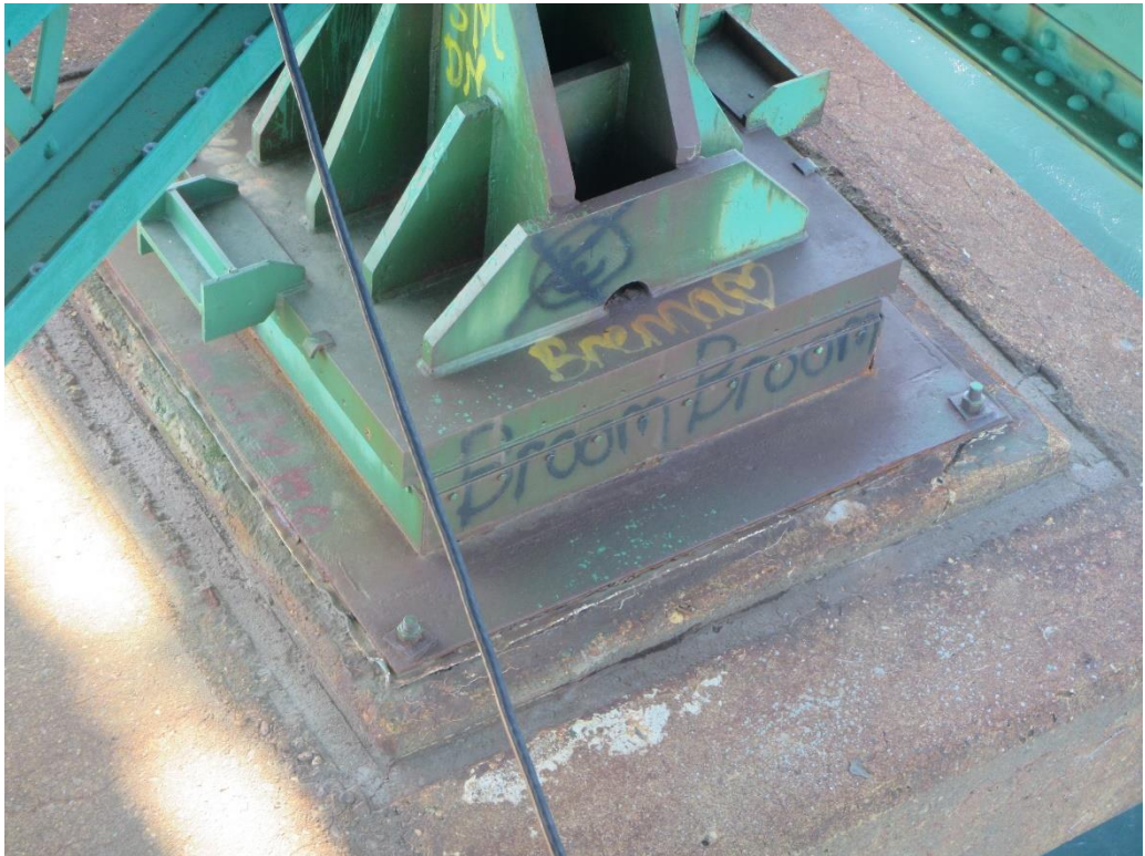
Figure 37: Pier 3 expansion bearing
