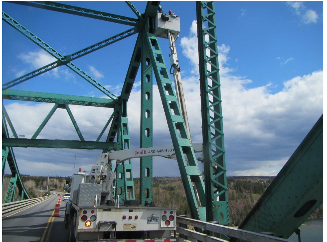
Figure 27: Example of specialized access (Jenik A-62) for under bridge inspection
