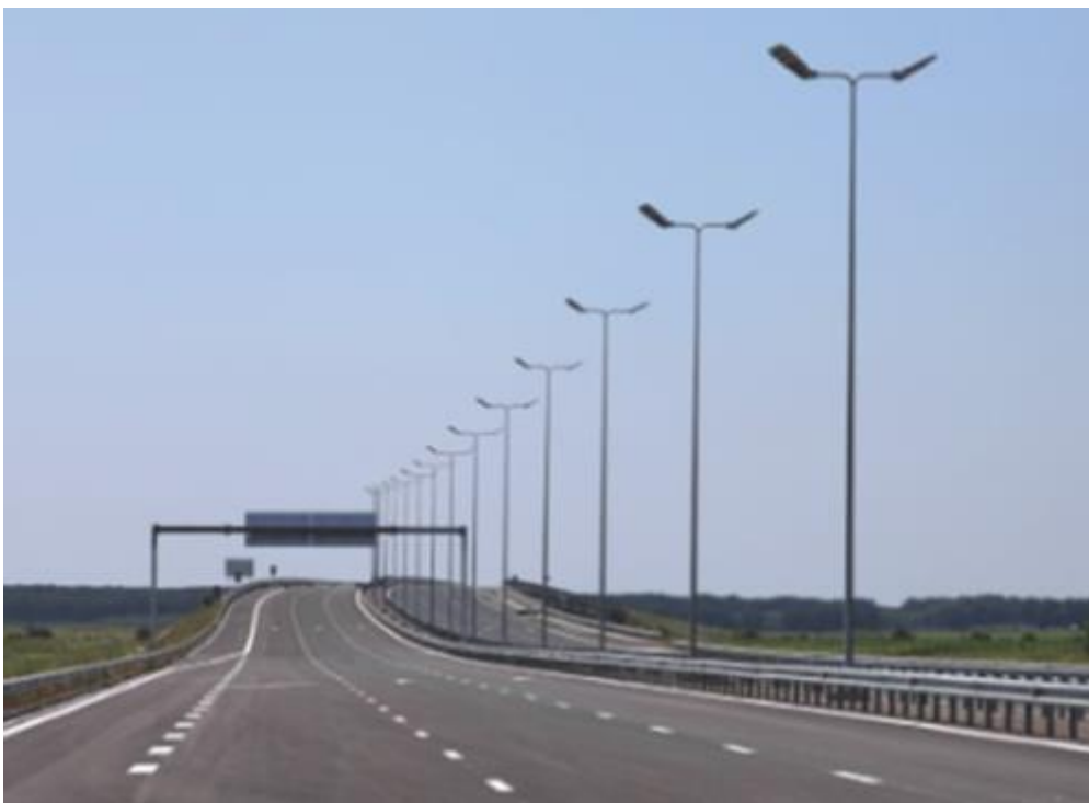
Figure 55: Typical offset roadway lighting suitable for edge or median installation. Source: www.holophane.com (n.d.).
