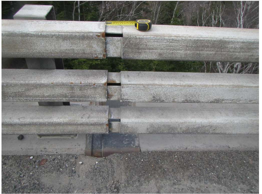
Figure 43: East abutment expansion joint
