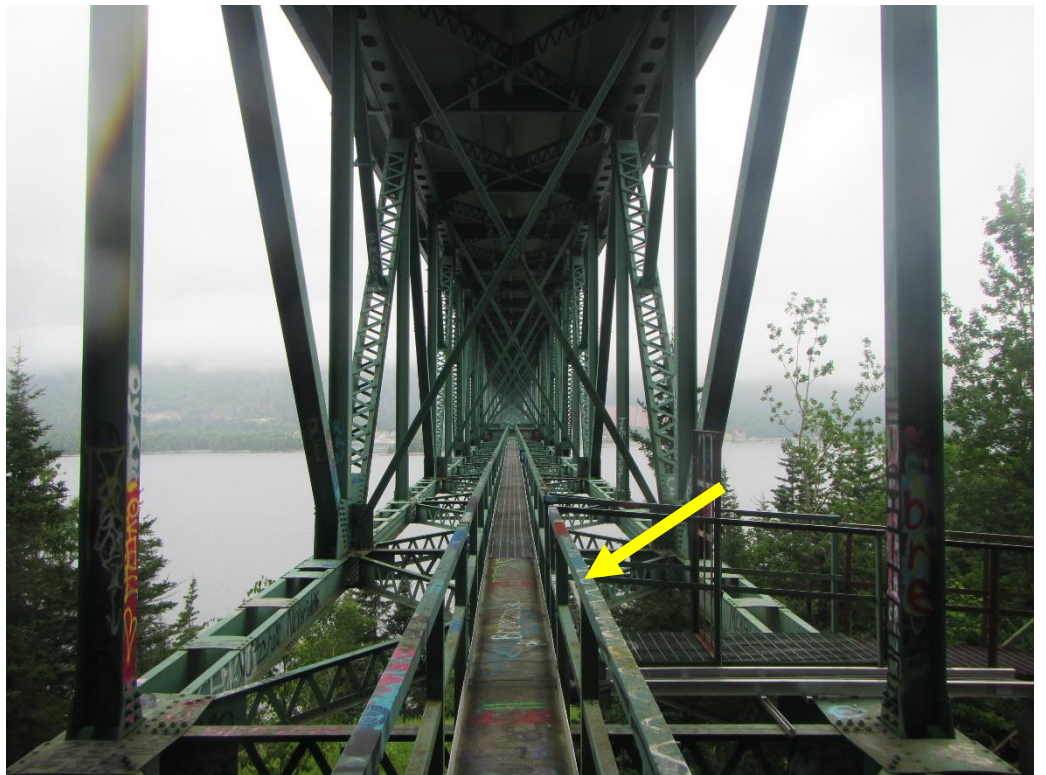
Figure 19: Underside view of approach truss showing longitudinal access catwalk
