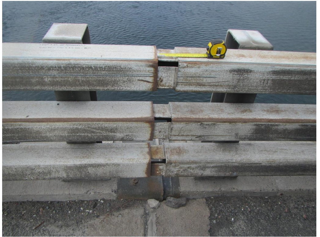
Figure 31: Pier 1 expansion joint at traffic barrier
