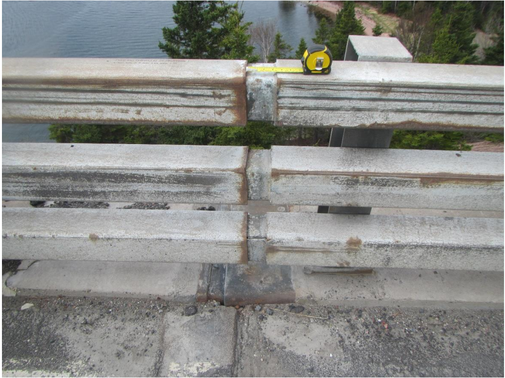
Figure 29: West abutment expansion joint at traffic barrier
