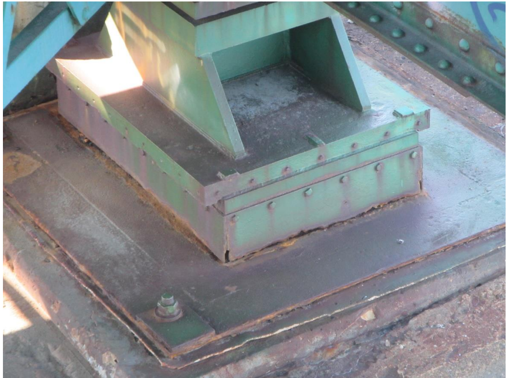
Figure 39: Pier 6 expansion joint at traffic barrier
