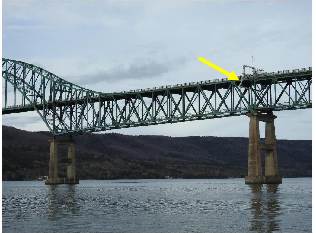
Figure 27: Example of specialized access (Jenik A-62) for under bridge inspection
