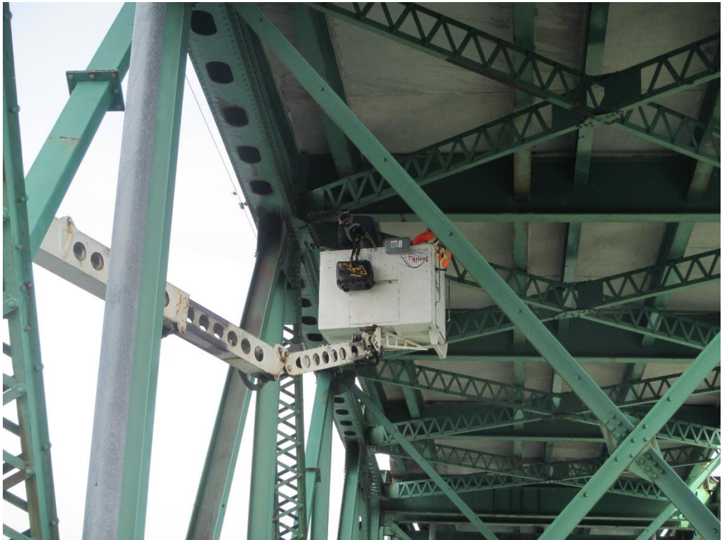
Figure 25: Example of specialized access (Jenik A-62) for under bridge inspection
