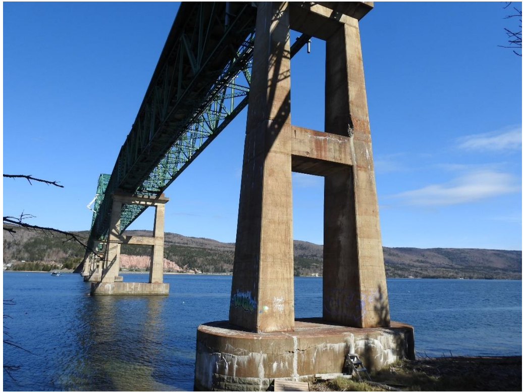
Figure 45: Typical substructure pier (Pier 7 shown)
