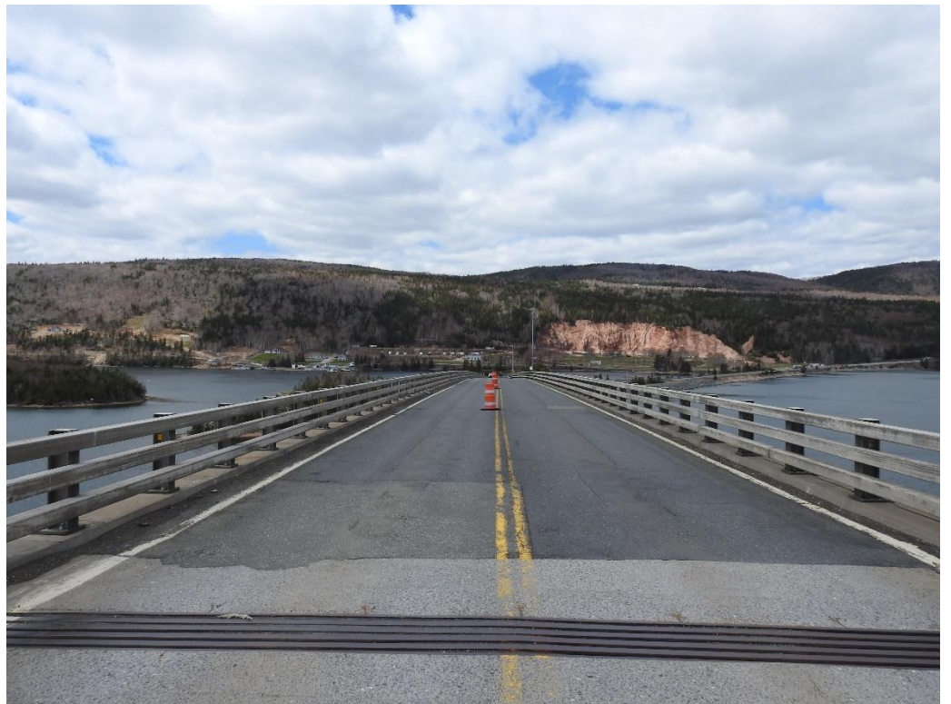
Figure 35: Pier 3 expansion joint at traffic barrier
