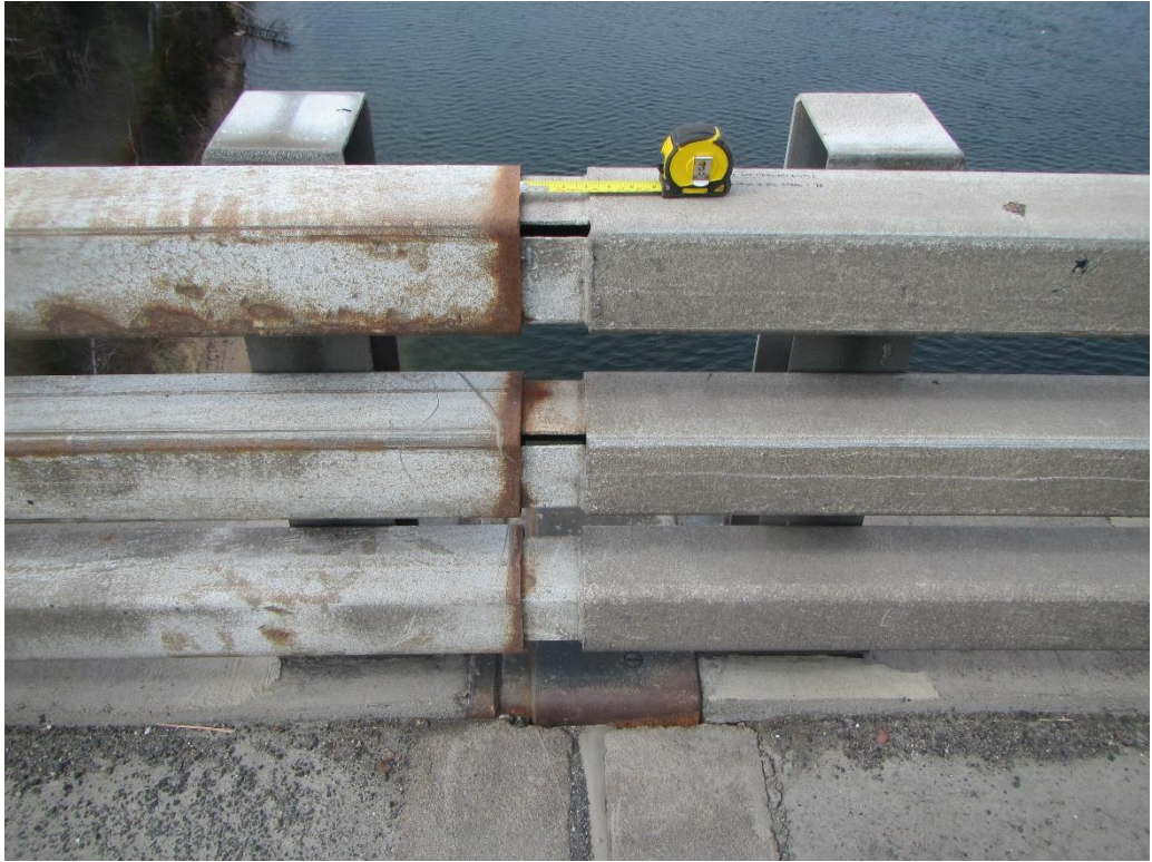
Figure 41: Pier 7 expansion joint at traffic barrier
