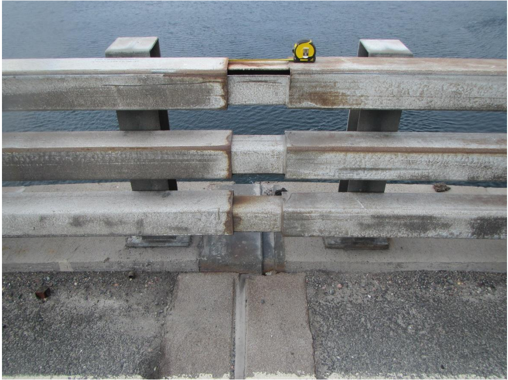
Figure 33: Pier 2 expansion joint at traffic barrier
