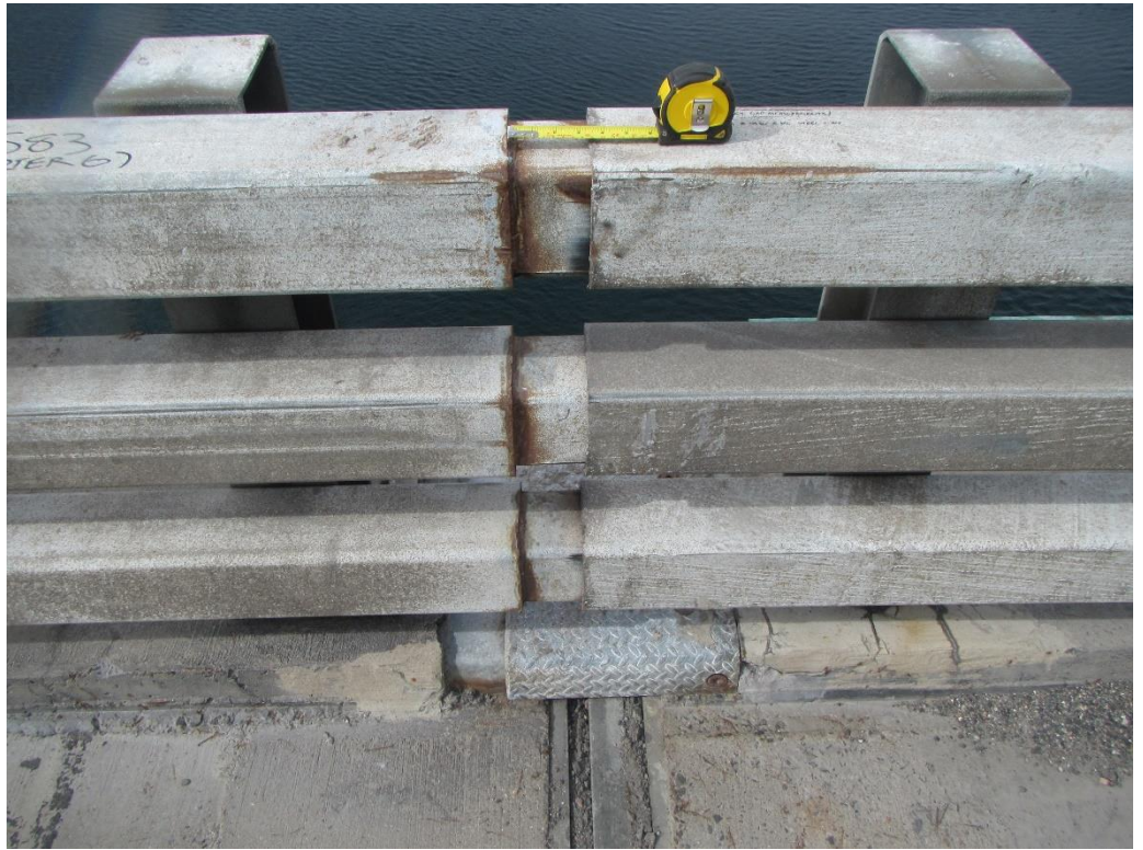
Figure 39: Pier 6 expansion joint at traffic barrier
