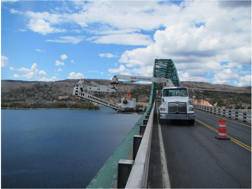
Figure 25: Example of specialized access (Jenik A-62) for under bridge inspection
