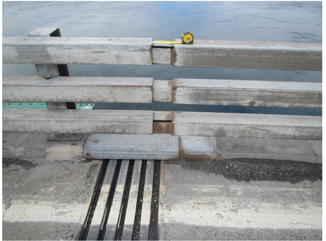
Figure 35: Pier 3 expansion joint at traffic barrier
