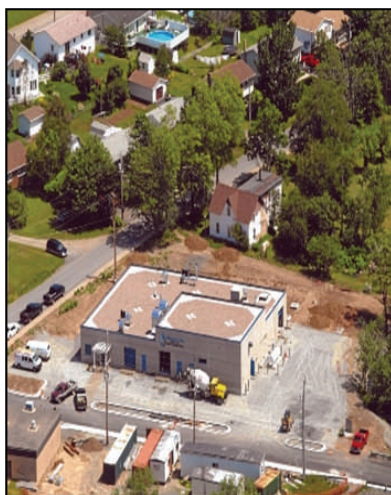
Aerial view of the treatment facility shows location in a residential area.
