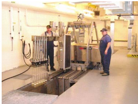
Medium Pressure, High Intensity UV lamps inactivate pathogens
