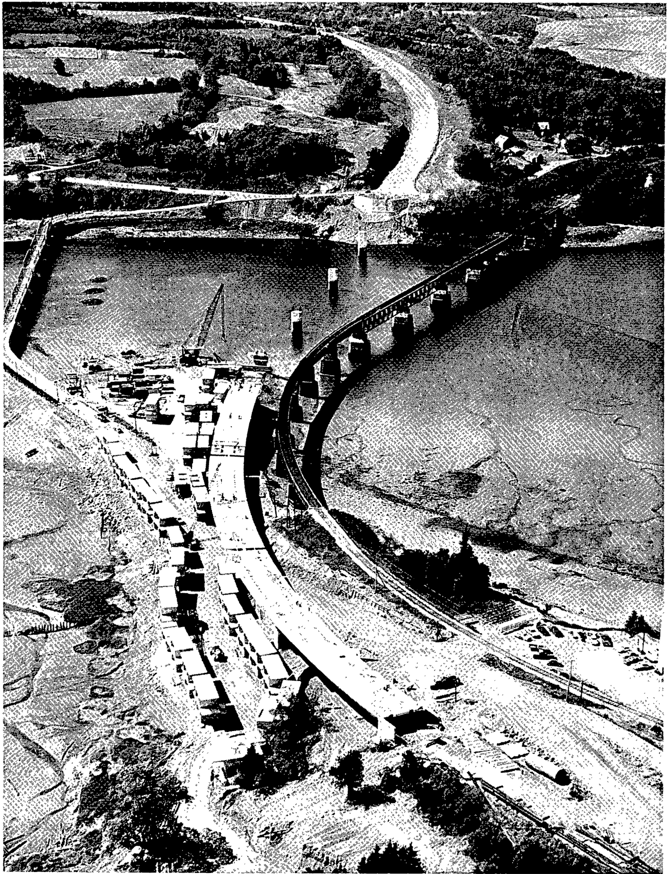
Frontispiece: Bear River Bridge and Highway 101 under construction.
