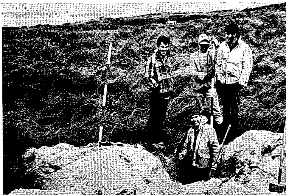
Figure 11. Location of benchmark buried under 4 feet of windblown sand between 1963 and 1971.
