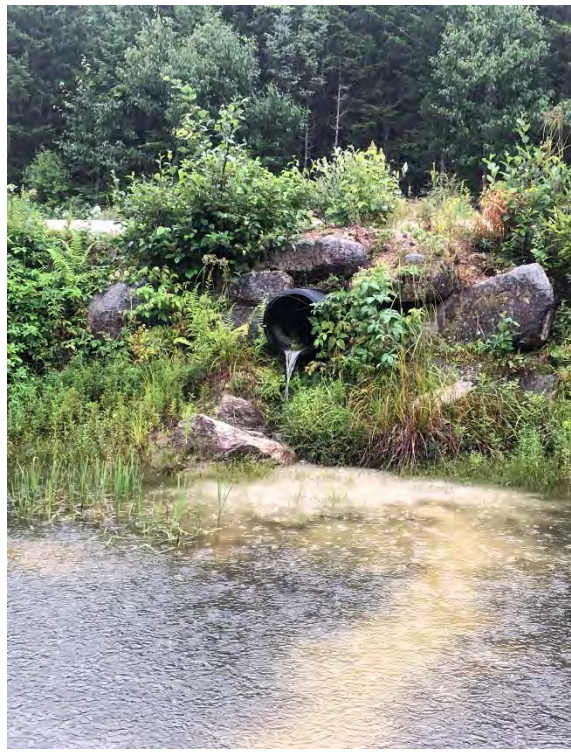
Photo 20: Pond1 culvert inflow
