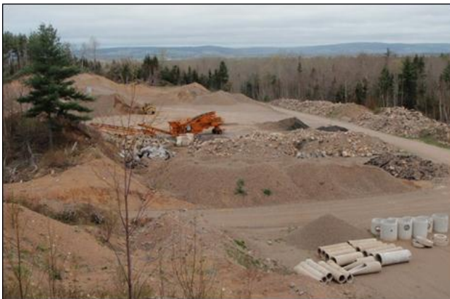
Photo 4.3: South pit, looking north.
