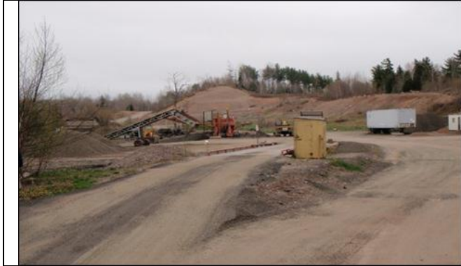
Photo 4.1: Central pit area with weigh bridge, crusher and aggregate stockpiles.
