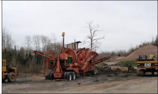
Photo 4.2: Central pit crusher.
