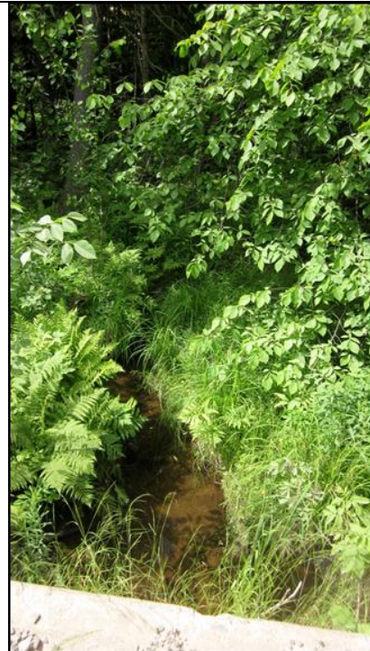
Plate 4: Watercourse on East side of culvert facing East
