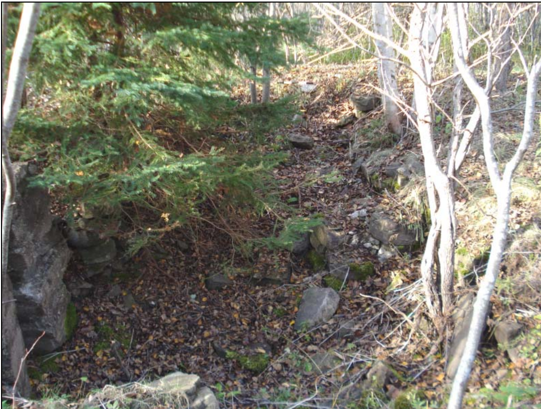
Plate 8: West end of Concrete Foundation 2.
