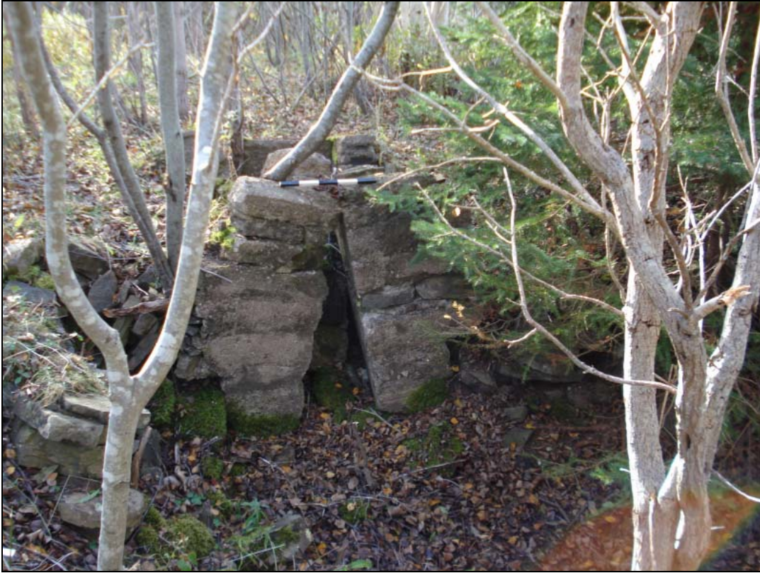
Plate 7: South end of Concrete Foundation 2.
