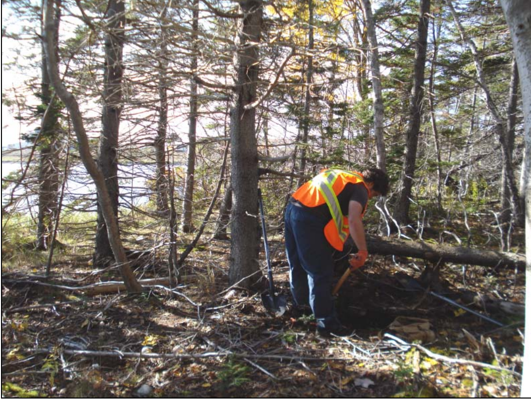
Plate 13: Railway crossing test pits.
