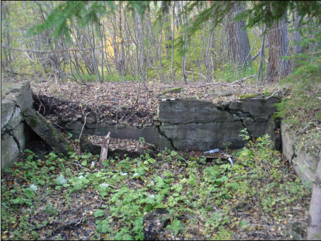
Plate 5: East side of Concrete Foundation 1.
