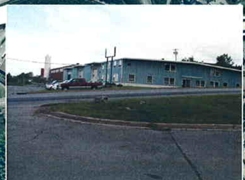
SITE FROM WRIGHT AVENUE SHOWING SIDE PARKING AND LOADING AREA. MARITIME PAPER IS IN BACKGROUND.
