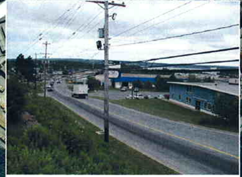
FROM WRIGHT AVENUE. PROPOSED SITE IS AT RIGHT OF PHOTO. GUILDFORD'S INC. (BRIGHT BLUE BUILDING) IS SHOWN IN BACKGROUND.
