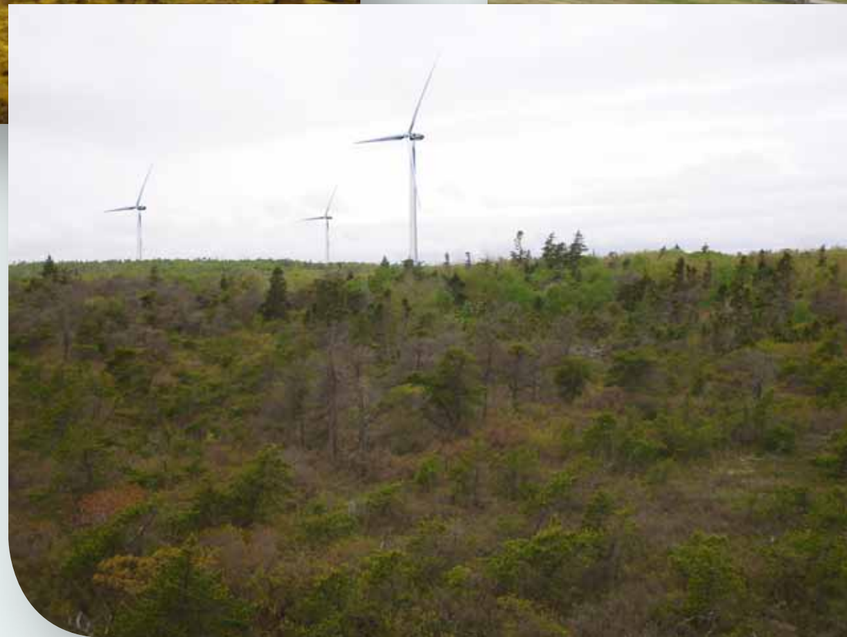
Photo IV: Looking SouthWest Into Project Site – Observation Platform on Chapel Gully Trail
