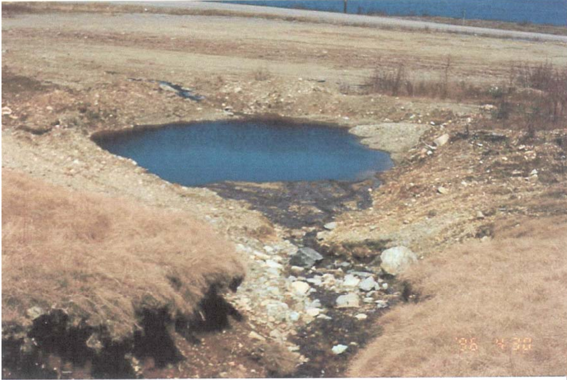
Photo 1: One of several settling ponds constructed at the Sheet Harbour Industrial Park as part of the storm water management plan infrastructure. Photo taken April 30, 1996.
