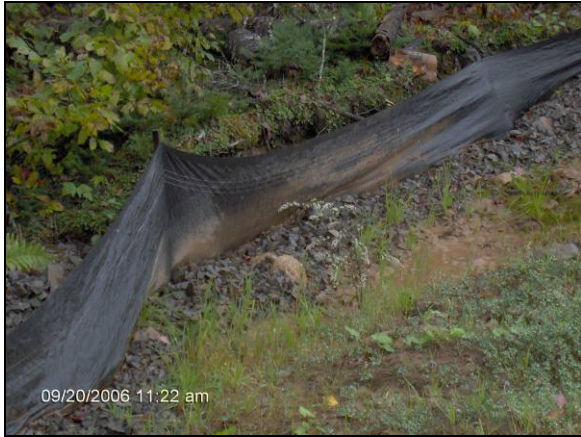
Photo 1. Silt control screens erected around the SW perimeter of the quarry
