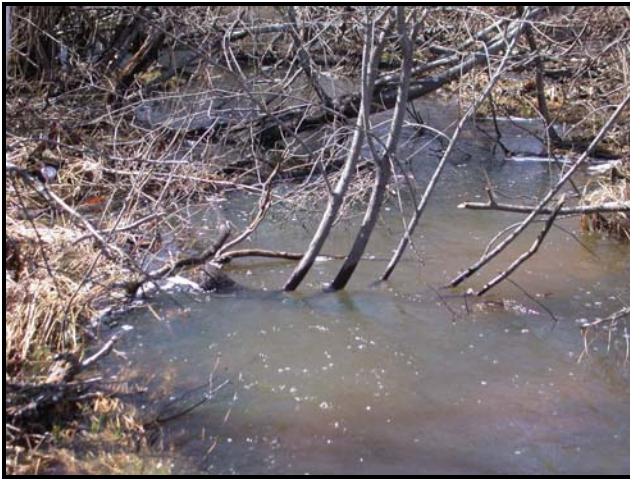
Photo 3 Looking Further Downstream of Culvert on Property Access Road – April 2005
