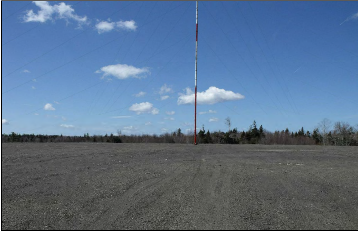
Plate 3: MET tower base and pad looking southwest.
