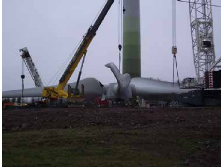
Photo 8. Hub and Blade Lift.
