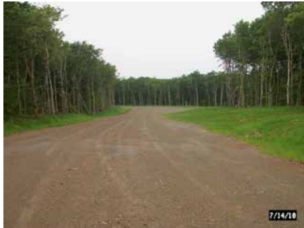
Photo 2. Example Access Road
