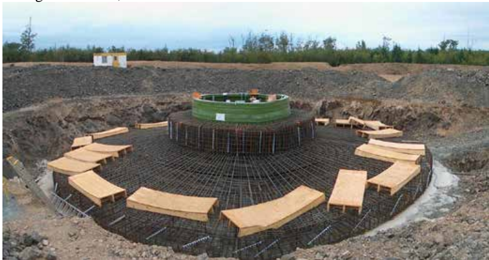
Photo 4. Typical turbine re-bar installation for the spread foot foundation.
