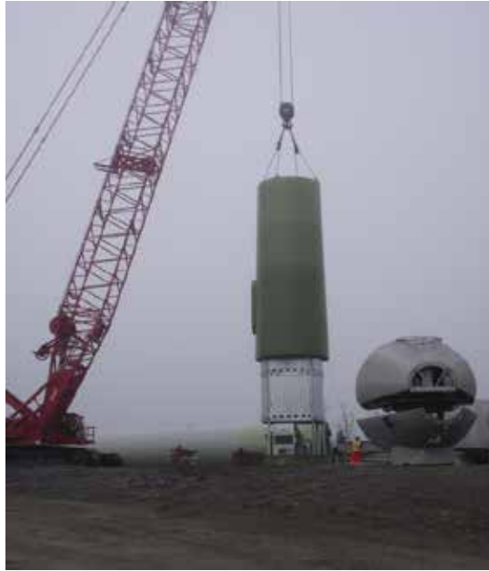
Photo 6. Tower section installation
