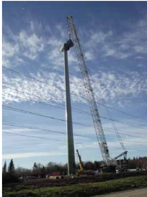
Photo 7. Nacelle Installation
