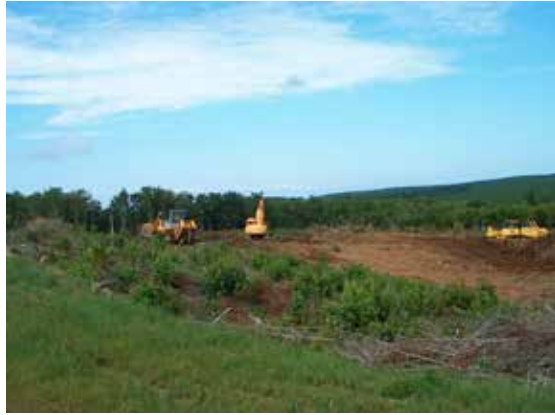
Photo 3. Typical clearing operations of a turbine site following timber removal
