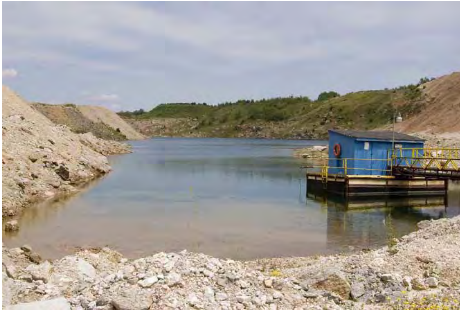
Photo 6.7-7: Settling Pond in Miller's Creek Quarry
