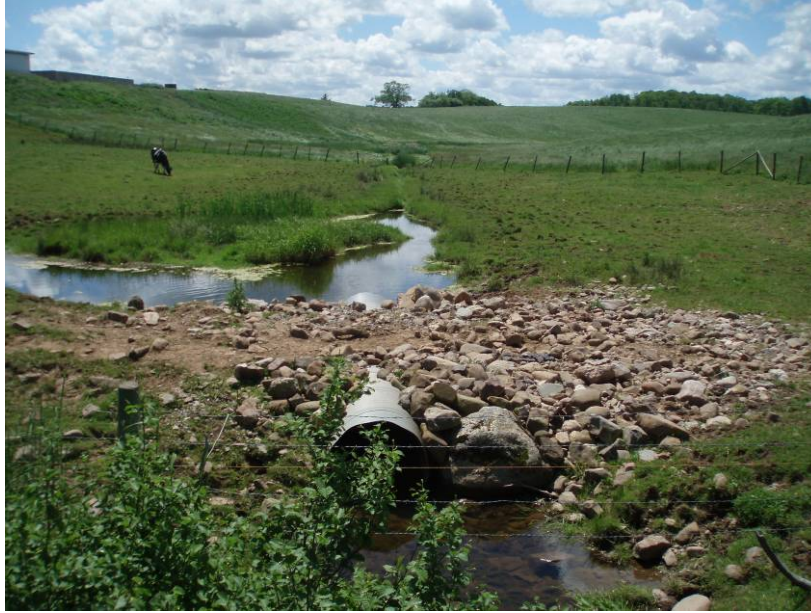
Photo 27: Shaw Brook downstream of Avondale Road, note instream habitat disturbance from trampling, improperly size culvert and excavation for cattle watering.
