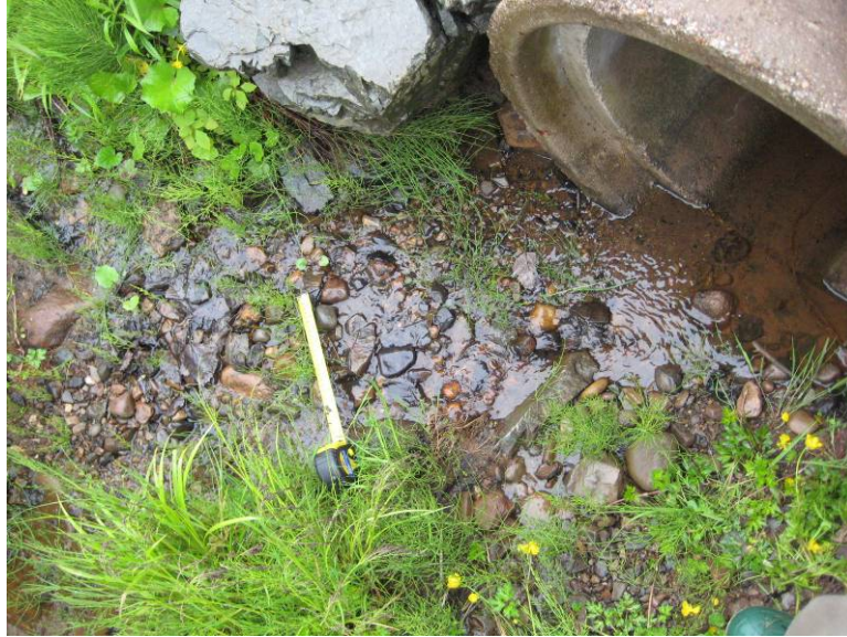
Photo 4.2.6: Flow conditions at SW-11 culvert inlet (June 11, 2009)
