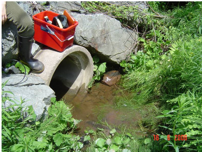
Photo 4.2.1: Flow conditions at SW-11 culvert inlet (June 6, 2006)
