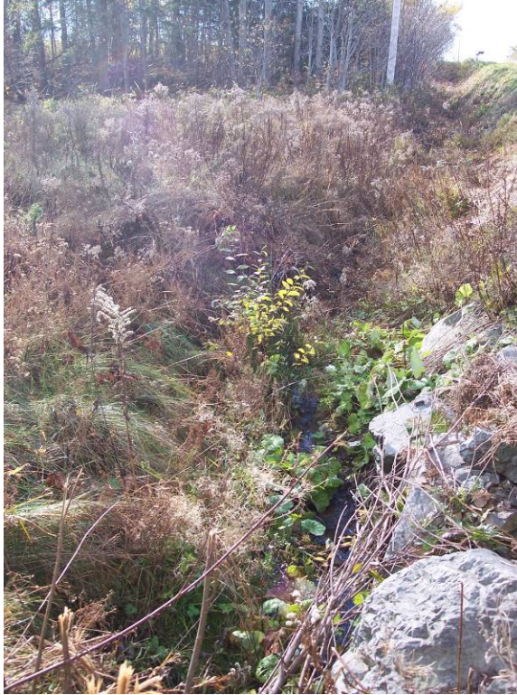
Photo 4.2.2: Flow conditions at SW-11 culvert inlet (November 3, 2006)
