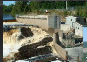
Morgan Falls Run of River Hydro Power Plant 1995
