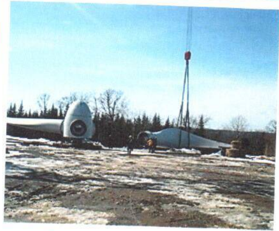
Figure 3: Assemble of Rotor for Watts Section Project (2011).
