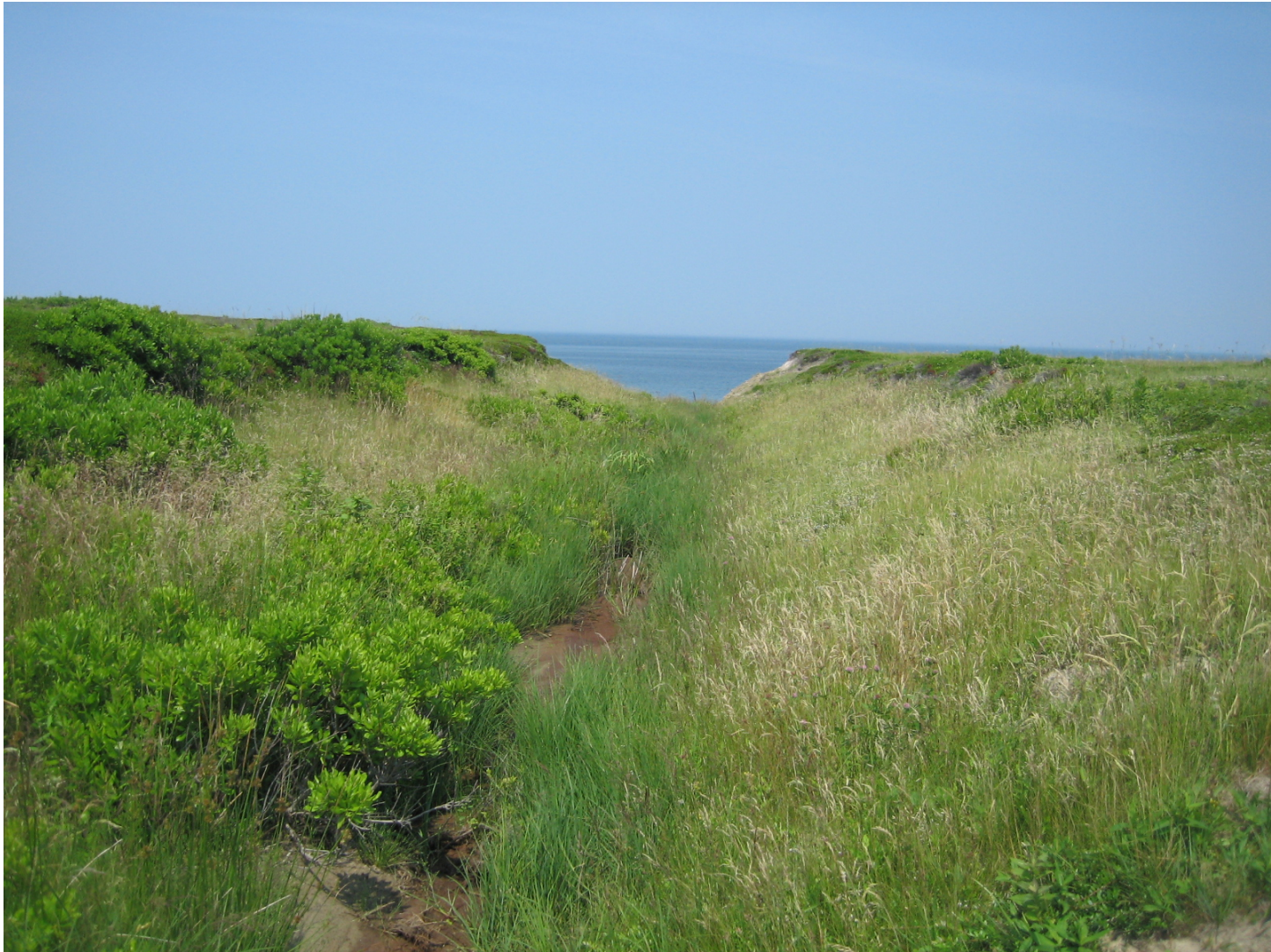
Plate 3 Outlet of drainage ditch west of Turbine #7
