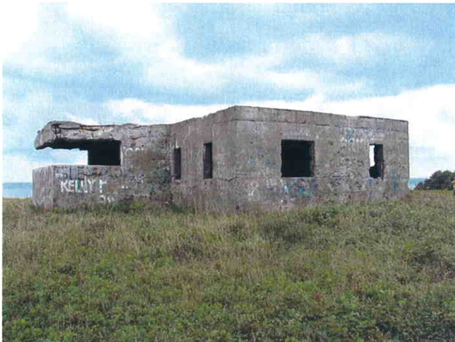
PLATE 2: North Head Forward Observation Post. Facing south.
