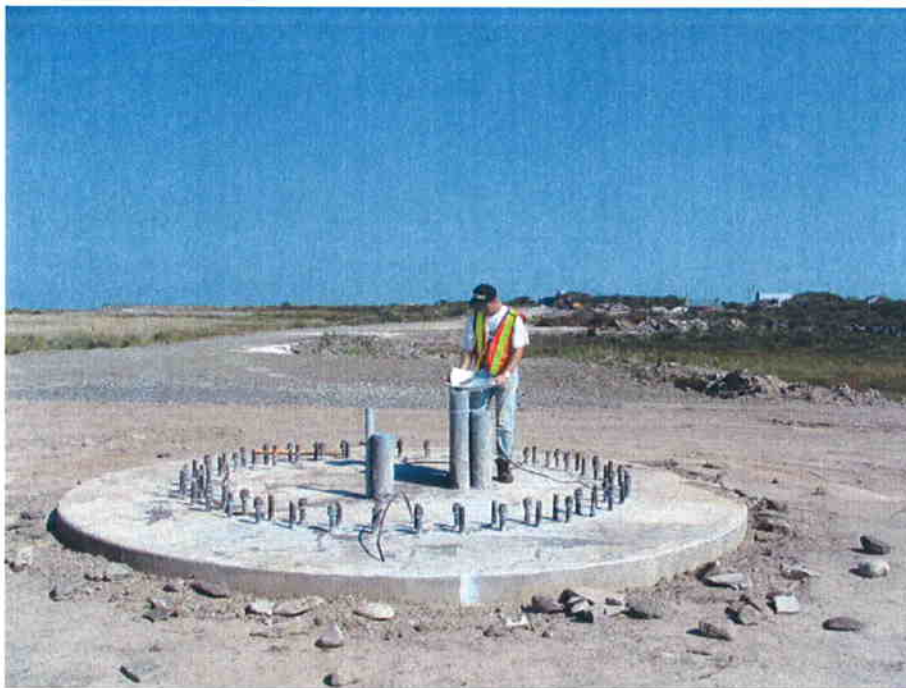
PLATE 4: New turbine base and access road at the 1-B Colliery site in Bridgeport. Facing northeast.
