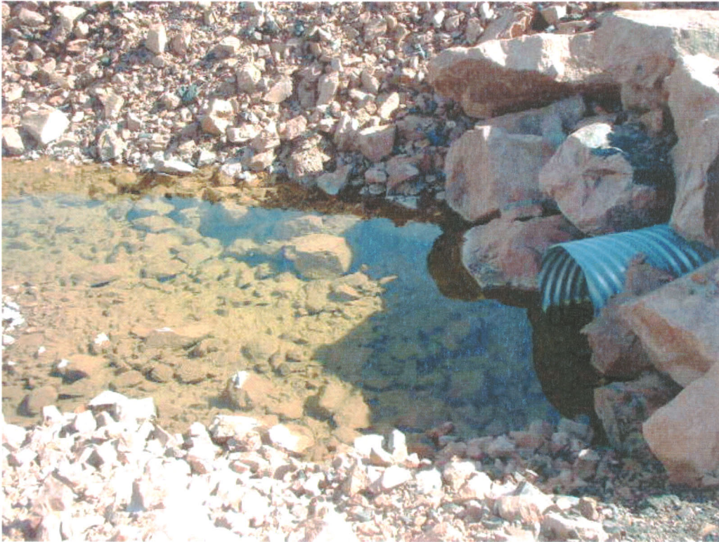
Photo 9 Drainage culvert inlet, August 2003
