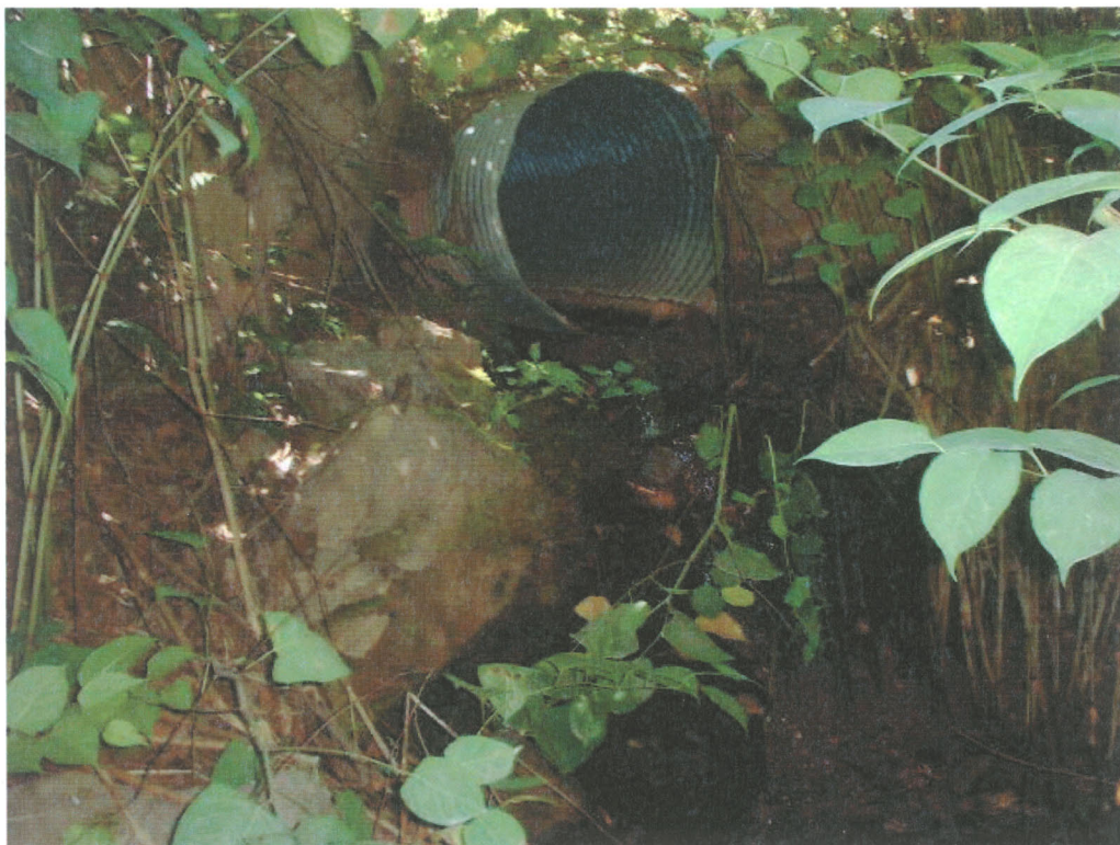
Photo 12 Stream crossing at Kemptown Road (downstream), August 2003
