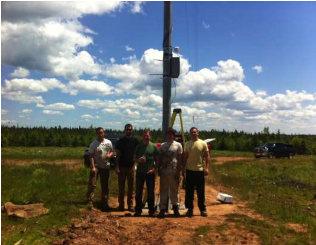
Figure 2.1 Technicians having just completed met tower construction at Kempton, June 2013
