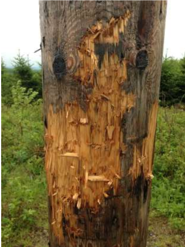
Figure 6.12 Power Pole at Dalhousie with Black Bear Markings, Spring 2013.
