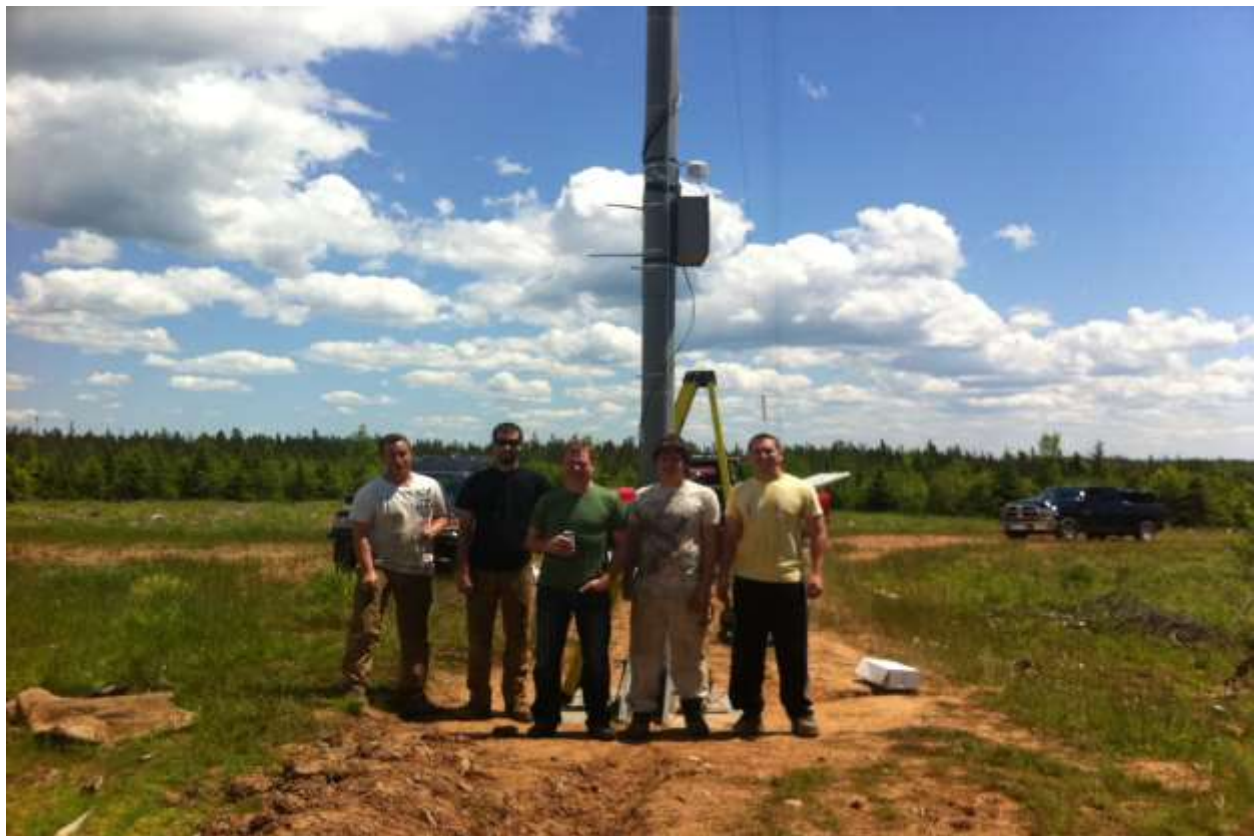
Figure 2.1 Technicians having just completed met tower construction at Kempton, June 2013
