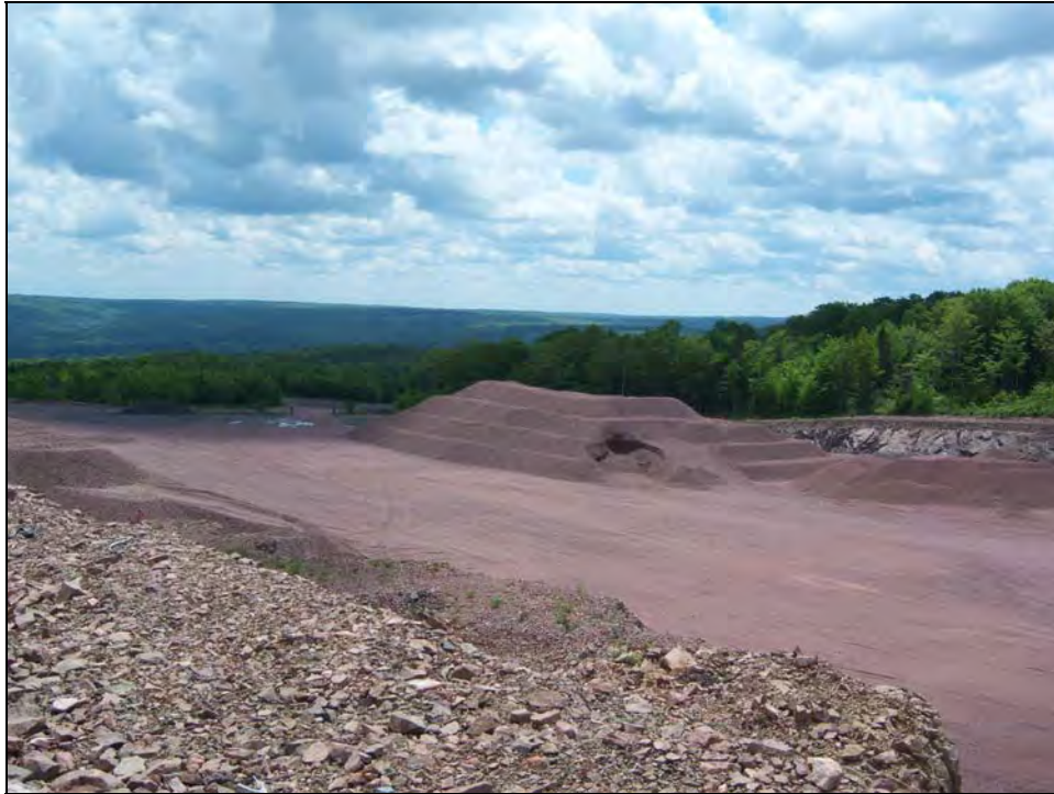
Figure 3. View of quarry towards entry gate in June 2013.
