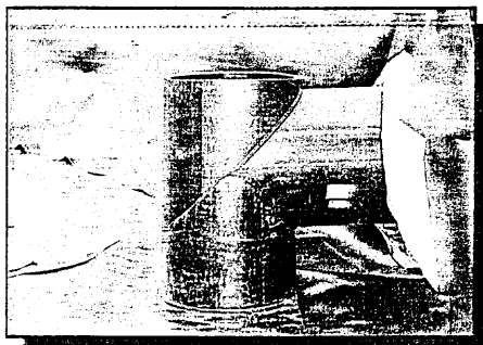
Over Flow Stand Pipe
