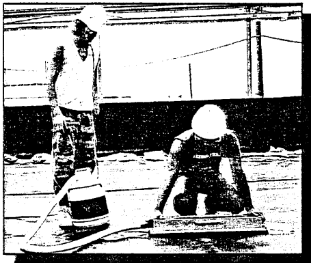
Liner seams are tested for leaks by vacuum, pneumatic, and tensiometer methods.
