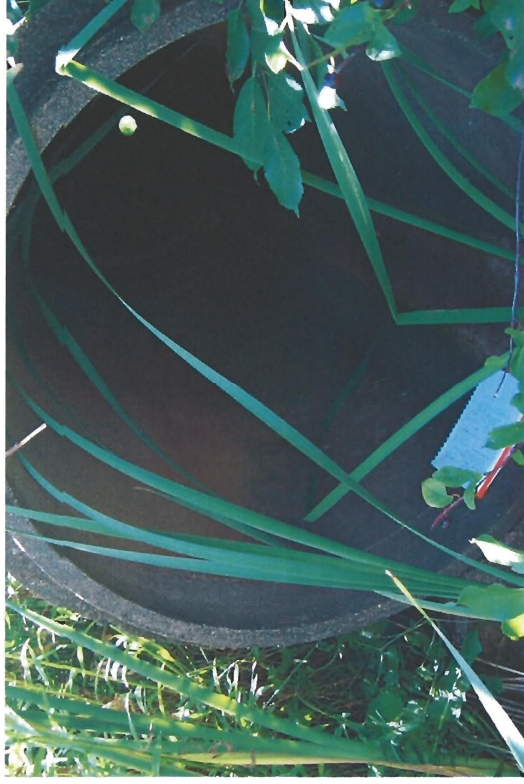
Photograph 4 – Un-named 0+275 Existing concrete culvert downstream side
