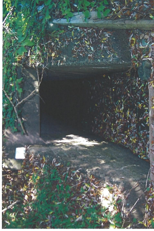
Photograph 48 – Existing structure under highway 104 (downstream of un-named 10+250) upstream side
