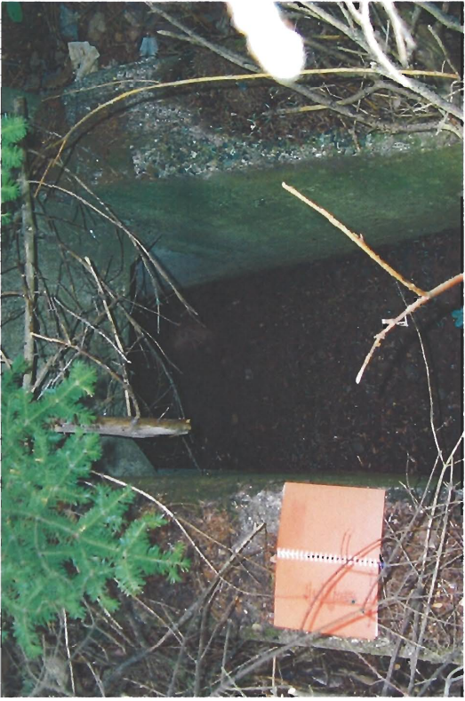
Photograph 53 – Un-named 13+600 Existing structure at proposed crossing, upstream side
