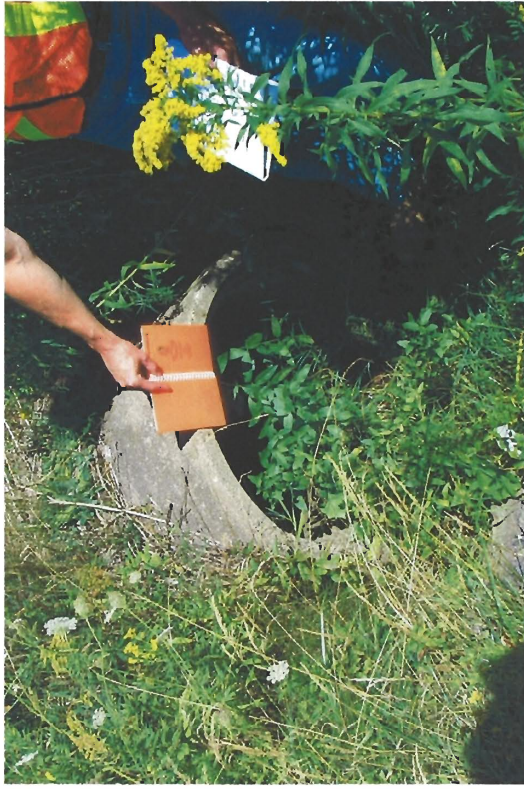
Photograph 3 – Un-named 0+275 Existing concrete culvert upstream side
