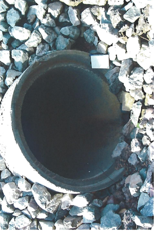
Photograph 50 – Existing structure under highway 104 (downstream of un-named 12+350) upstream side
