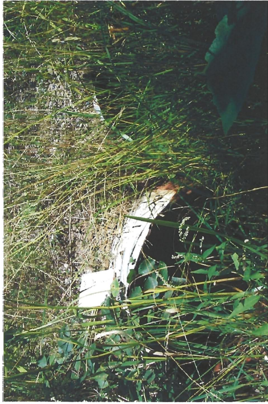
Photograph 11 – Un-named 2+075 Existing culverts upstream side
