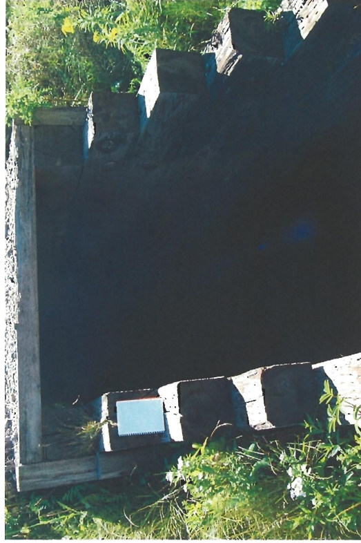
Photograph 8 – Un-named 0+600 to 0+850 Existing timber culvert downstream side at 0+750
