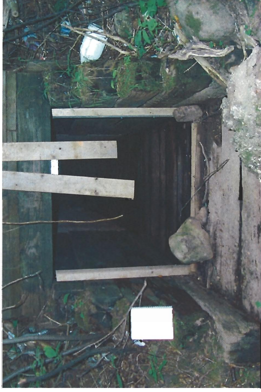
Photograph 52 – Existing structure under secondary road (downstream of un-named 12+350) upstream side
