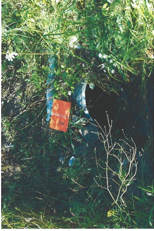
Photograph 26 – Un-named 4+150 Culvert under driveway upstream of crossing location
