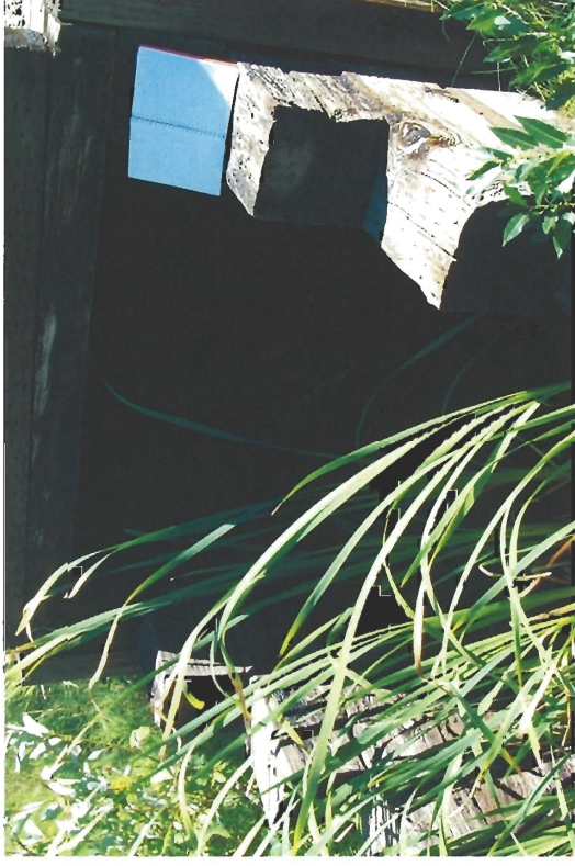
Photograph 10 – Un-named 1+400 Existing timber culvert upstream side
