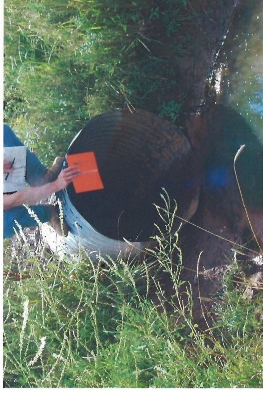
Photograph 36 – Existing Structure at Beech Hill Road (downstream of un-named 6+950) downstream side
