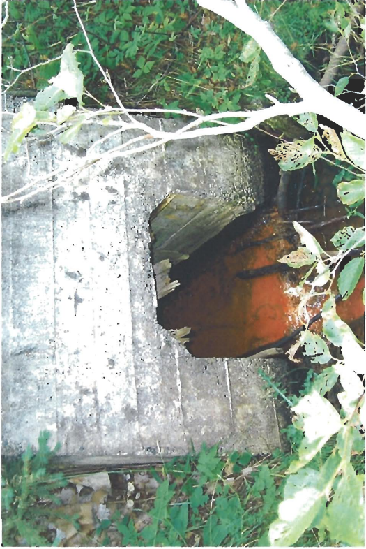
Photograph 57 – Un-named 14+580 Existing structure at proposed crossing, downstream side
