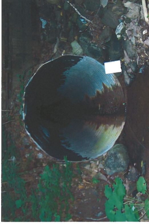
Photograph 46 – Existing structure under highway 104 (downstream of un-named 10+250) downstream side
