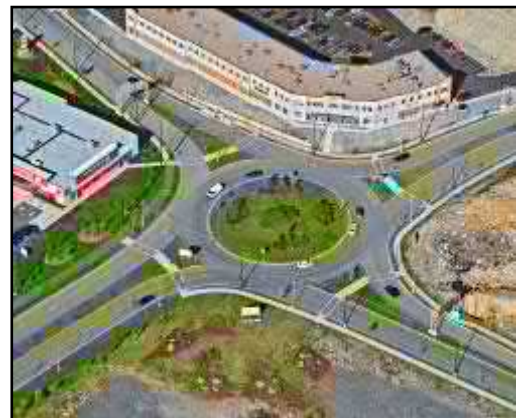
Photo 1 Typical Roundabout (Photo provided by NSTIR)
