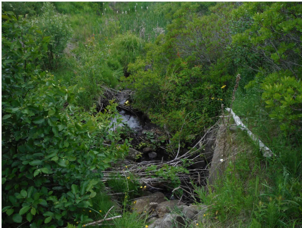
Photo 5.3 WC3a concrete culvert
