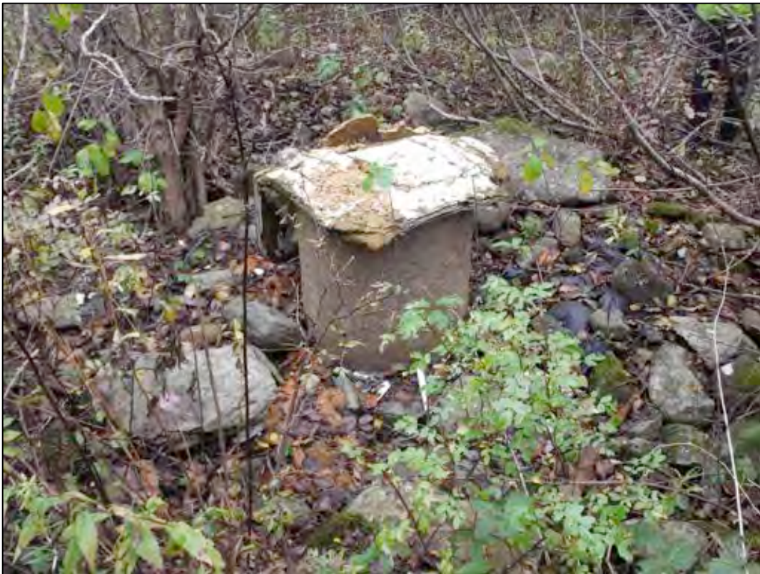
Plate 22: A concrete crotch well presumed to have fed the abandoned house to the north. Looking northeast.
