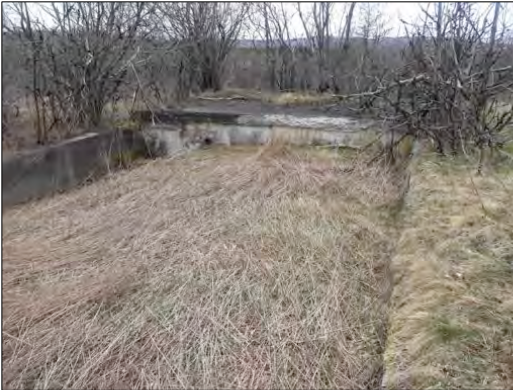
Plate 16: A concrete foundation remaining from the 1968 barracks complex, looking north. Please note that this photo was taken during geophysical survey work in April 2016, prior to undergrowth regeneration in the spring.
