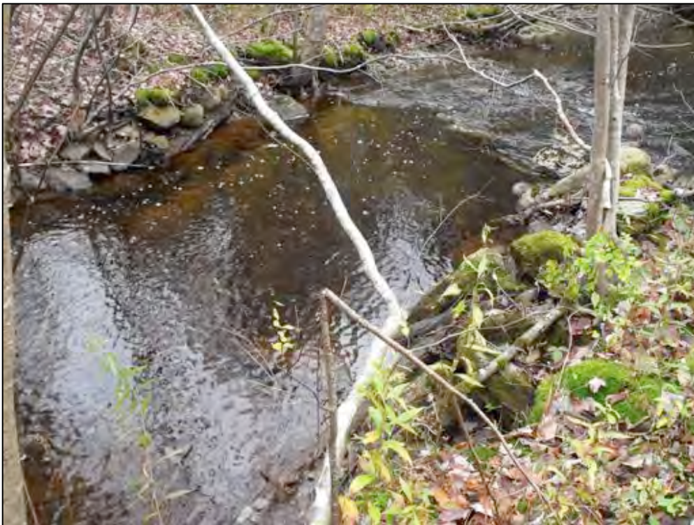
Plate 10: The two remaining edges of a stone dam across Seely Brook, looking south.
