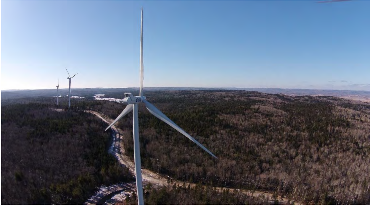
1 Martock Ridge Community Wind Project. Turbine 1 in foreground, looking south
