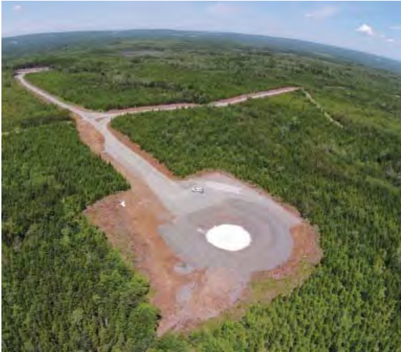
Road completion and foundation excavation
