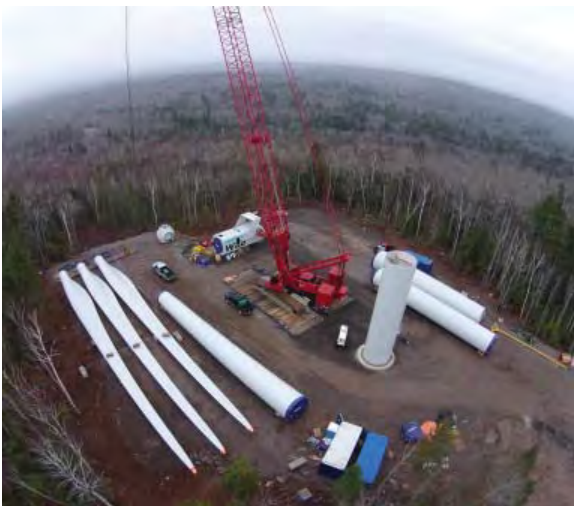
All components on site with crane
