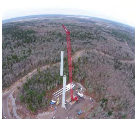
Tower components left into place
