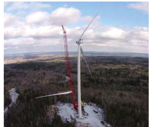
Last blade lifted into place
