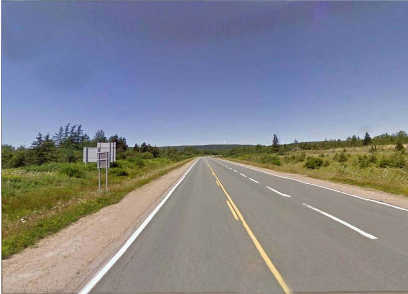
View of Project from Highway 101
