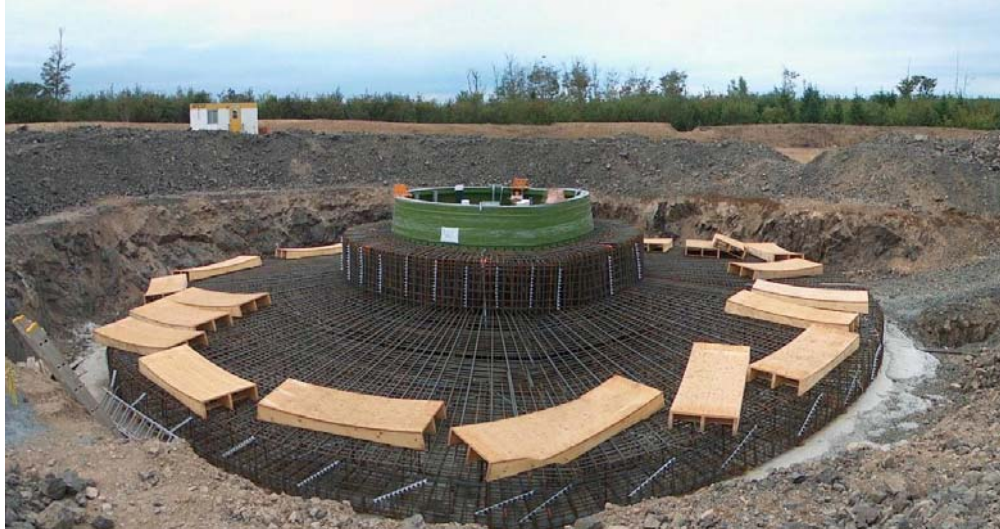
Photo 2. Typical turbine re-bar installation for the spread foot foundation.
