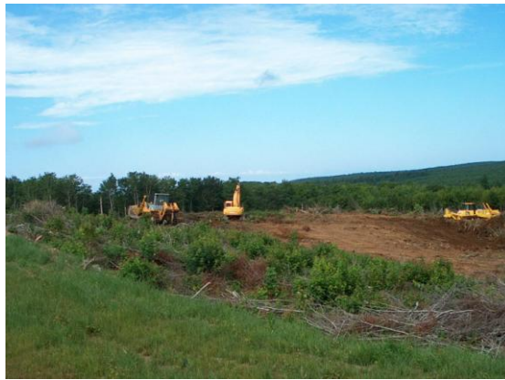
Photo 1. Typical clearing operations of a turbine site following timber removal
