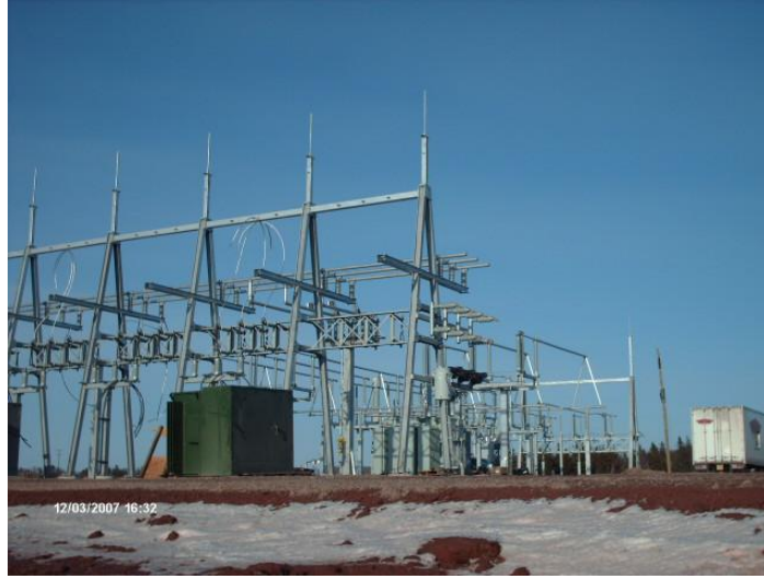
Photo 4. Typical substation under construction with 4 collection system circuits.
