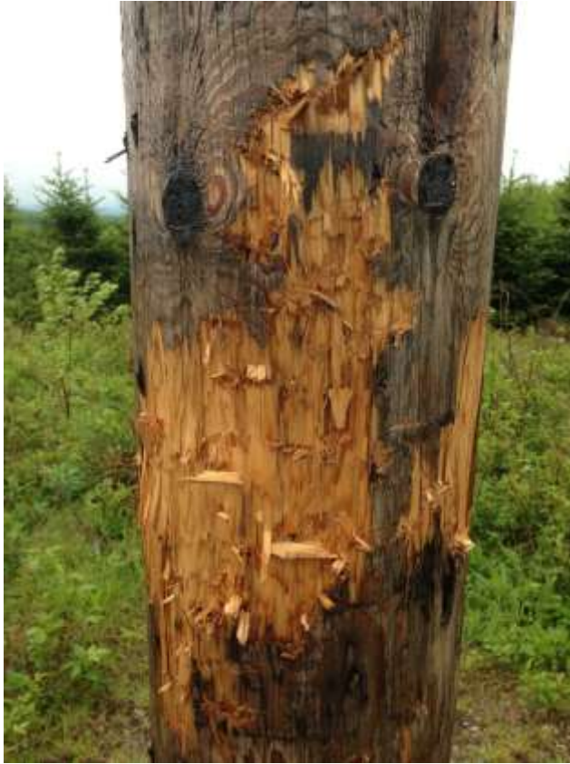
Figure 6.8 Power Pole at Dalhousie with Black Bear Markings, Spring 2013.
