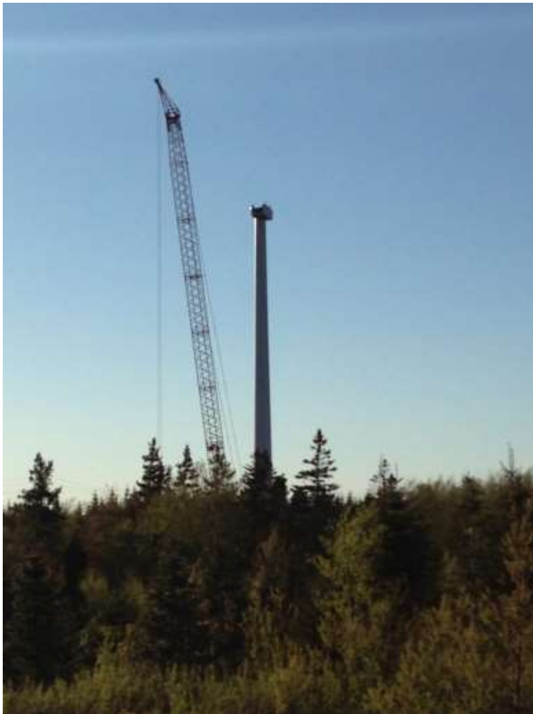
Figure 6.5 Turbine Tower Erected with Crane Ready to Hoist the Blade Assembly
