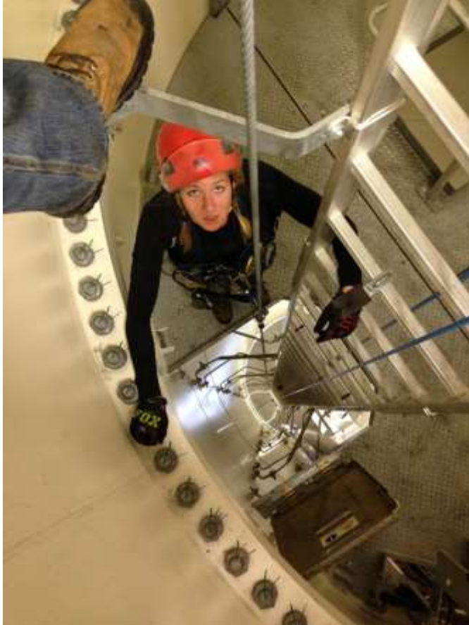
Figure 2.2 Employee in safety harness climbing down the ladder in GE turbine.
