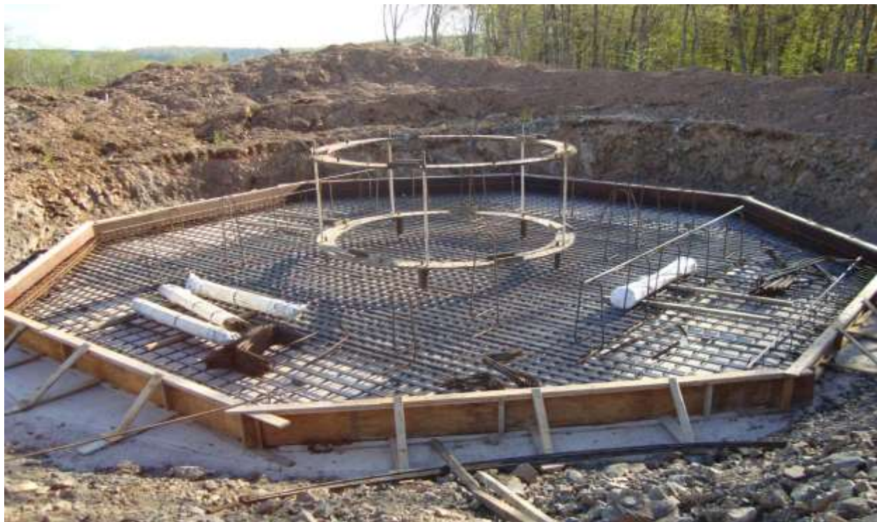
Figure 6.2 Foundation Partially Complete with Frames and Rebar in View
