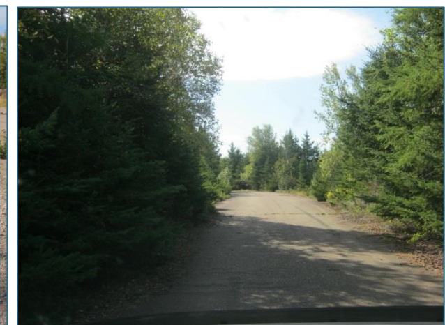
Photo 6 Paved Portion of Access Road
