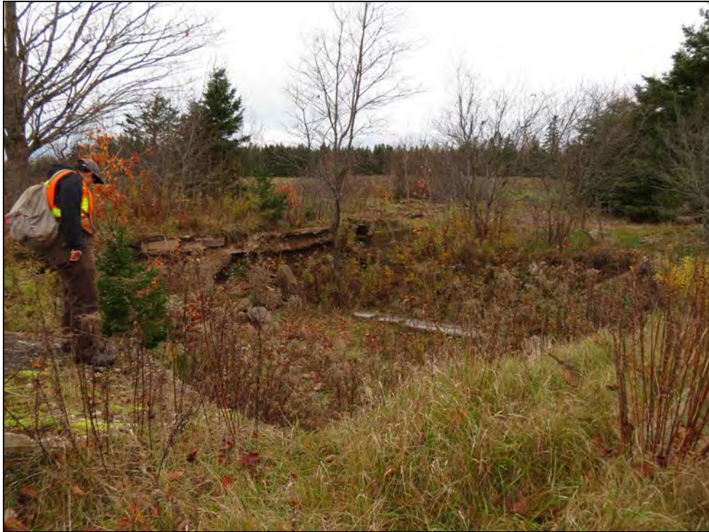
PLATE 8: Inspecting the concrete foundation of a demolished house, facing northwest. November 6, 2016.
