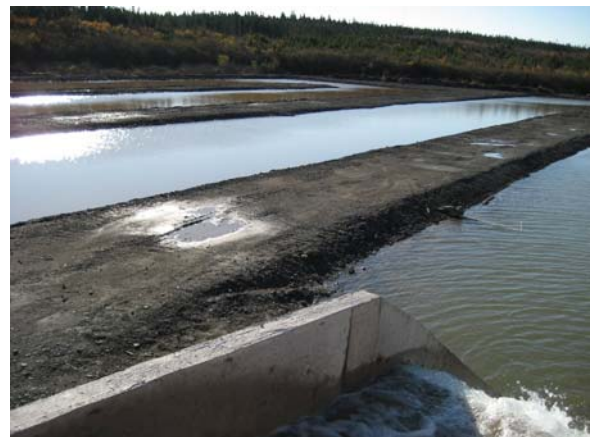
Aeration in the sedimentation basin through cascading the mine water
