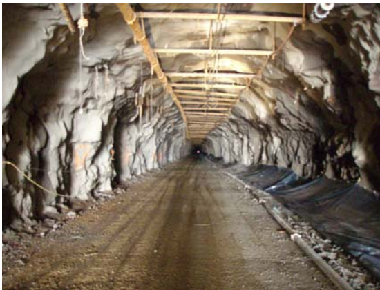
Drill and Blast Section
