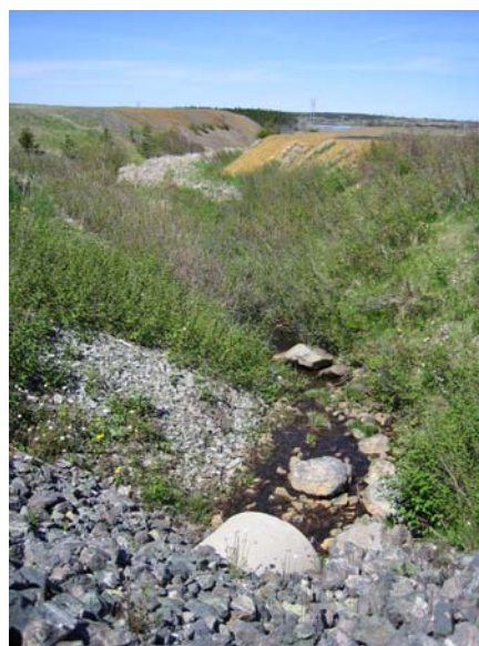
The central drainage channel passing between the two waste rock piles is a perfect water filtration system for surface runoff
