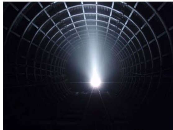
Tunnel Boring Machine Section
