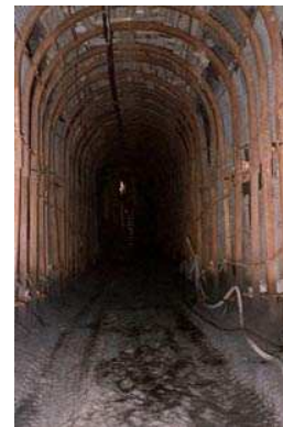
Donkin Mine Tunnel
