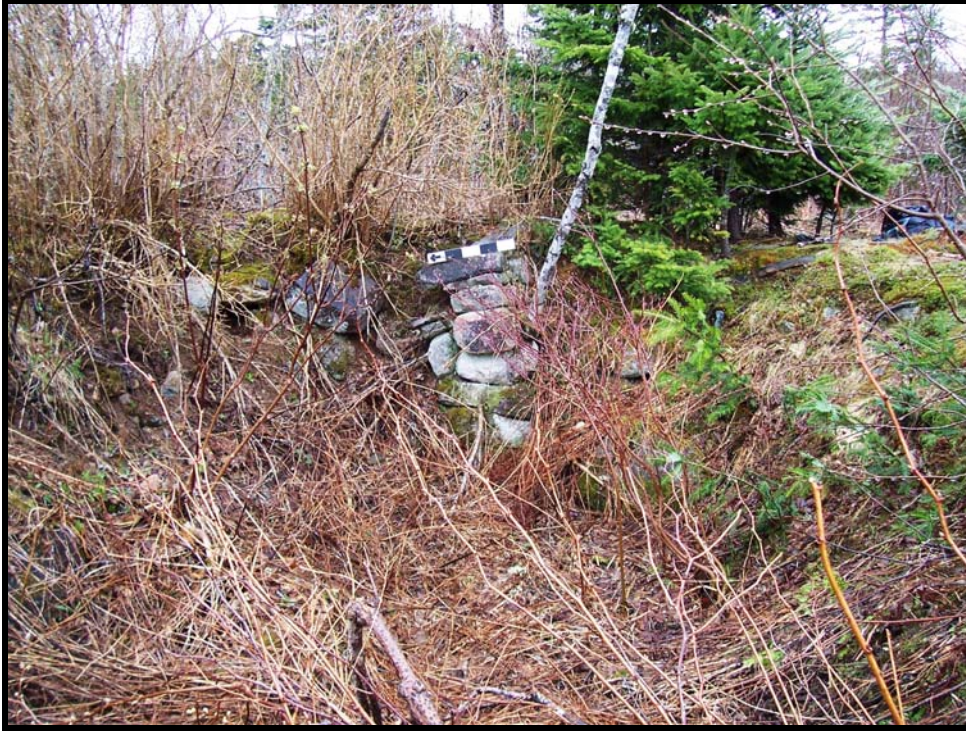
Plate 3: John Arthur foundation, near proposed turbine P1-40.
