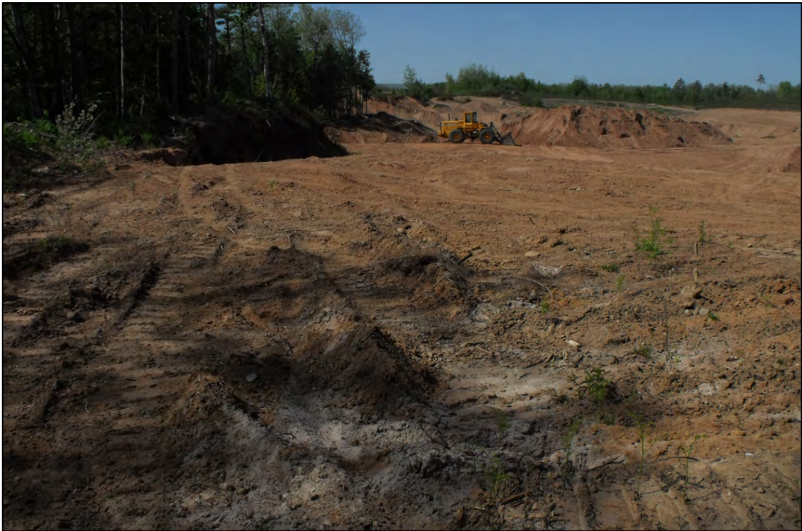
Plate 2: Approximately half of the existing pit, looking west.
