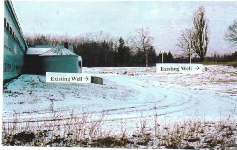
Photo #3. The nearest water wells located west of the active extraction area and the composting site. View west from active extraction area.
