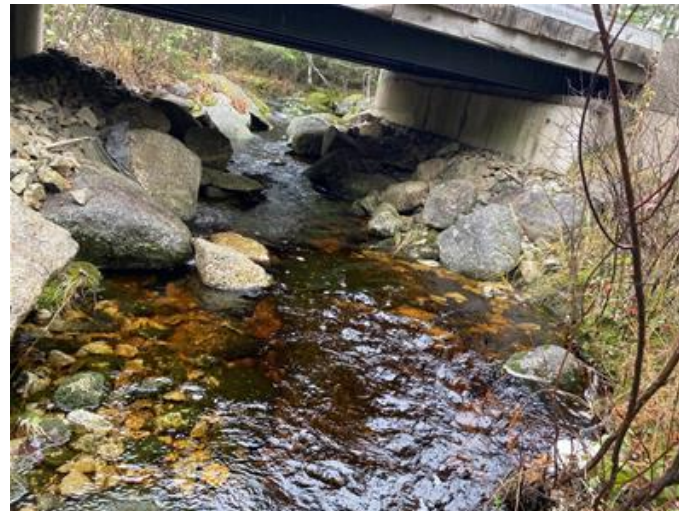
T2 November 1, 2022 at road crossing (bridge) of PDA
