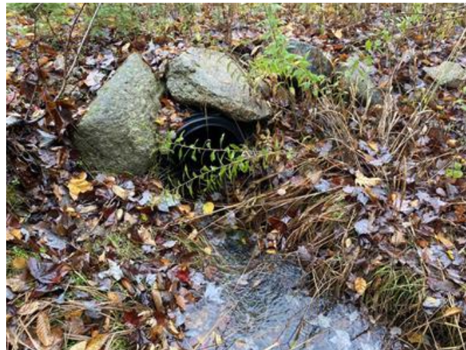
T1 October 19, 2022 upstream at road crossing (culvert) of PDA
