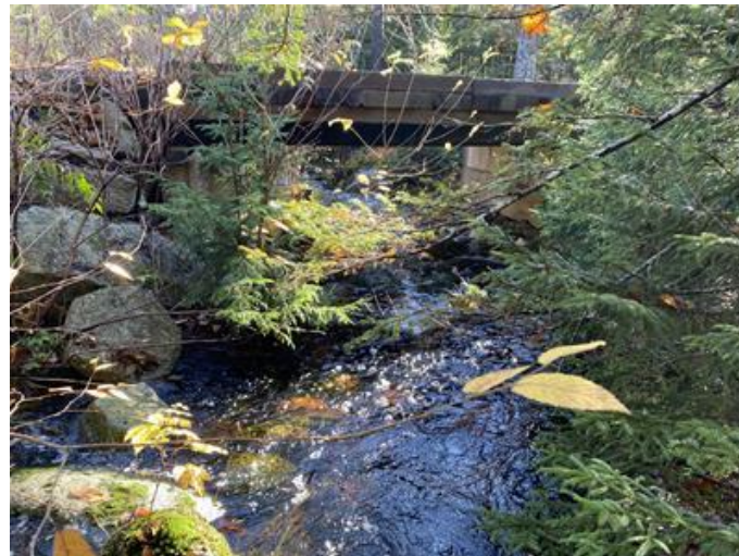
T2 October 20, 2022 at road crossing (bridge) of PDA
