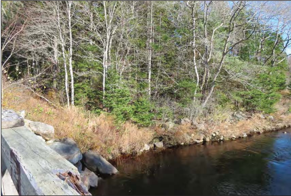
Plate 7: Morgan River crossing; facing east. November 13, 2015.
