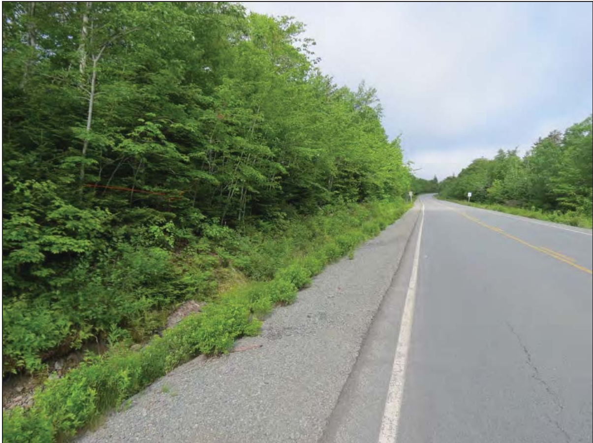
PLATE 1: The beginning of the Haul Road Option 2 alignment off Highway 224. The orange flagging tape denotes the alignment. Facing west. June 23, 2016.
